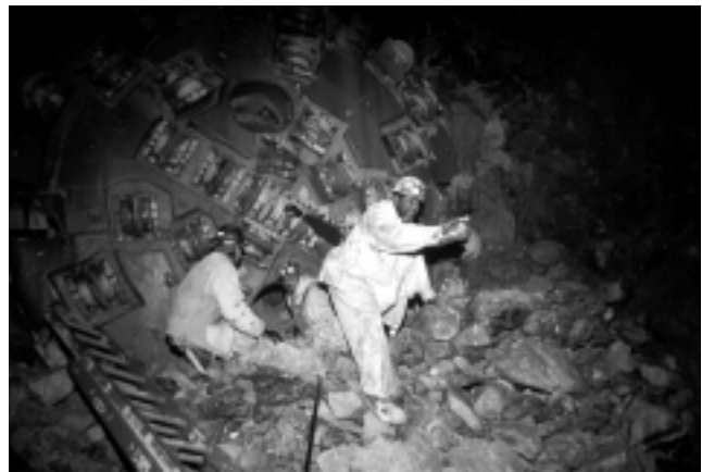
MetroWest Tunnel mining completed – October 27, 2000
