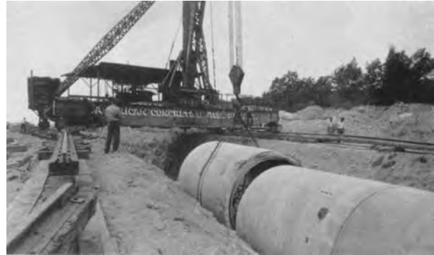
1946 laying Hultman Aq 138" RCP
