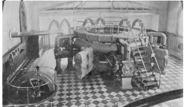
Corliss Spider – Installed in 1873 at Hope Pump Station, Providence RI, it had 5 steam cylinders, 5 pump cylinders and pumped 5 MGD
