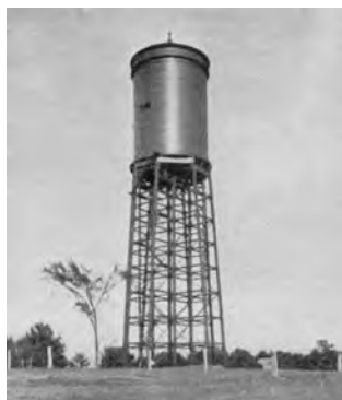
1905 East Providence RI Cast iron tank
