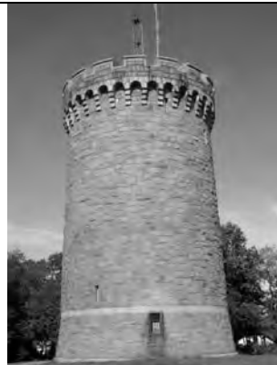
1902 Forbes Hill Standpipe, Quincy MA
