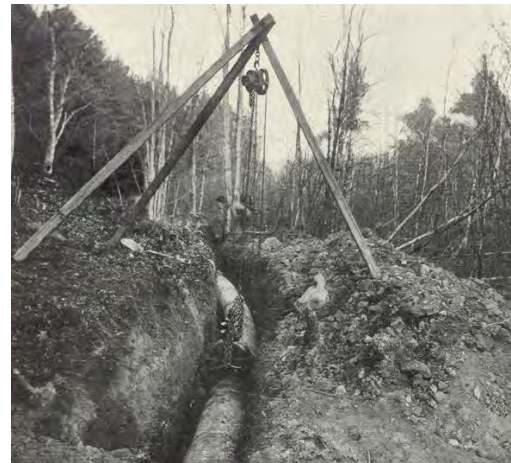
1916 14” wood stave pipe and valve, Pembroke NH
