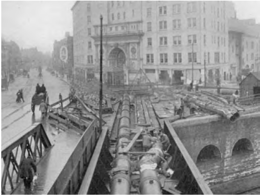
1912 pipe relocation for Boston subway, the original “Big Dig” for Boston
