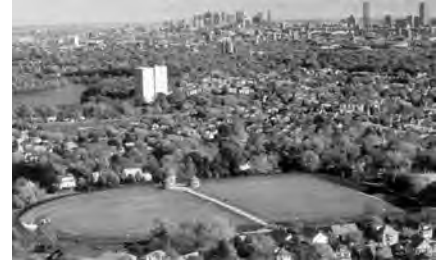
Modern day covered reservoir
