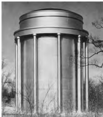
1963 Stamford CT standpipe featuring pillars
