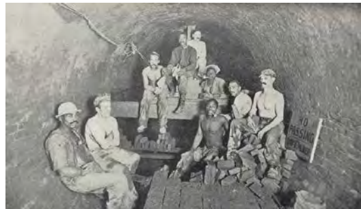
1908 Gloucester MA pipe tunnel – men working in pressurized tunnel
