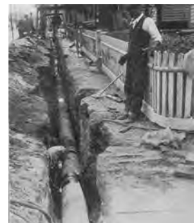
1927 welding steel pipe
