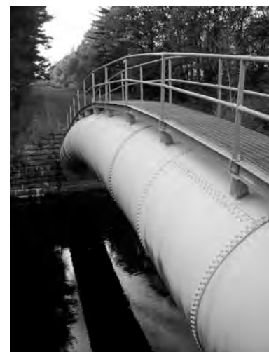
1903 Weston Aqueduct 84” steel self-supporting pipe bridge
