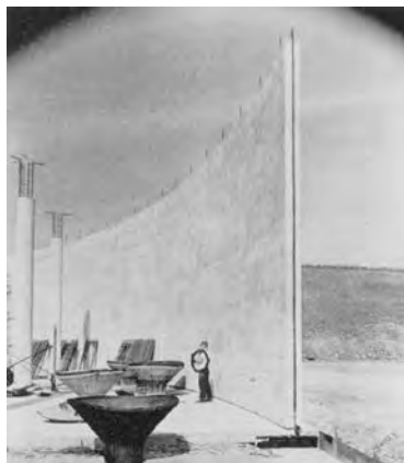
1959 Precast wall sections with integral waterproof core
