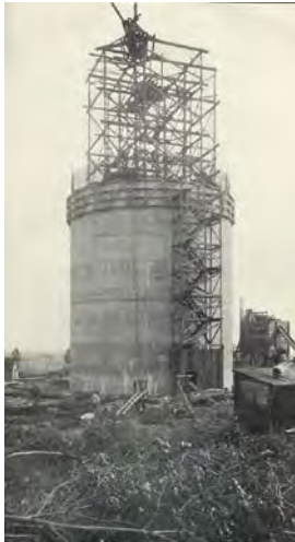
1906 Casting in place in lifts of several feet
