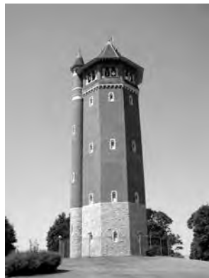
1895 Lawrence Tower, MA, AWWA Historical Landmark
