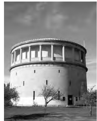
1921 Park Circle Standpipe, Arlington MA
