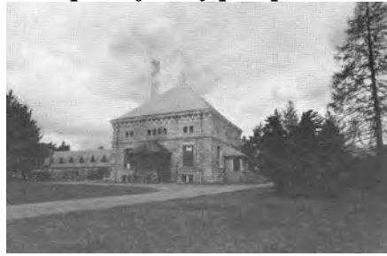
Quitticas Pump Station, New Bedford MA, AWWA Historical Landmark
