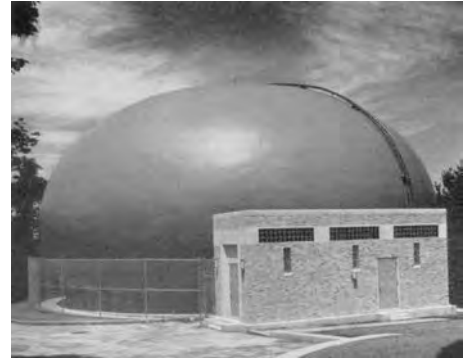
1938 Brookline MA – First spheroid tank in New England, it was chosen to protect against wind damage
