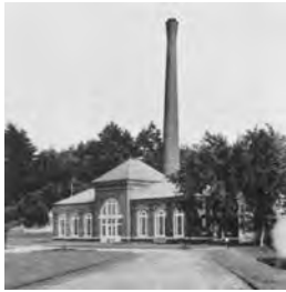
Snow Pump Station, Nashua NH, AWWA Historical Landmark
