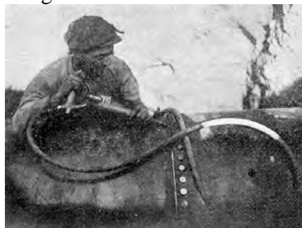
1924 caulking lockbar pipe
