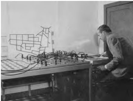
1951 early version of McIroy Pipe network analyzer
