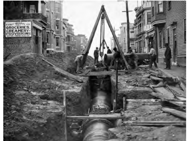
Pipe rigging at the site using chainfalls
