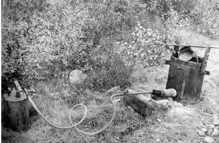
Kerosene fired lead melter for making pipe joints
