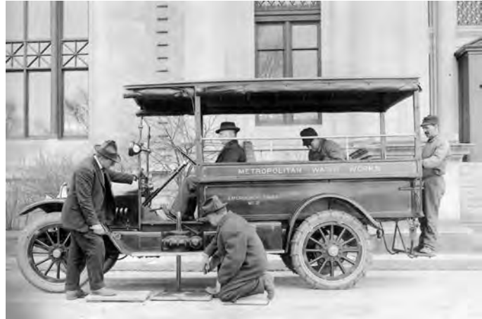
1919 MDC Emergency truck with valve operator mounted beside driver's door
