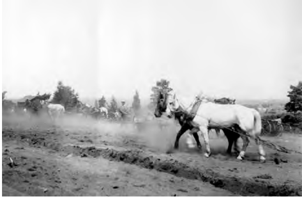
Horse drawn scrapers for grading
