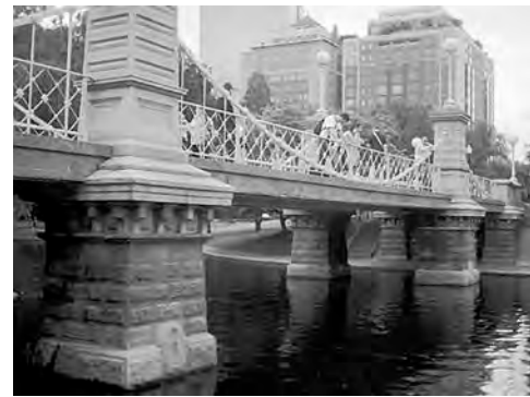
One of Herschel Clemens lesser known civil engineering projects was the design of the small suspension bridge in Boston's Public Gardens, an ASCE Landmark
