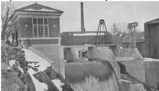
1925 Waterville ME hydroelectric power station with water supply pumping done by generated power
