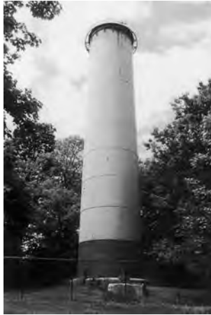
1881 Oldest steel standpipe, Dedham MA (now demolished)
