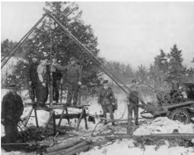
1933 Driving a tubular well
