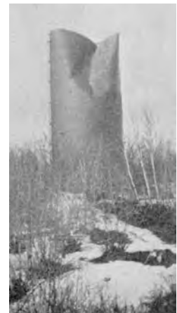
1921 Bath ME Failure of open top tank
