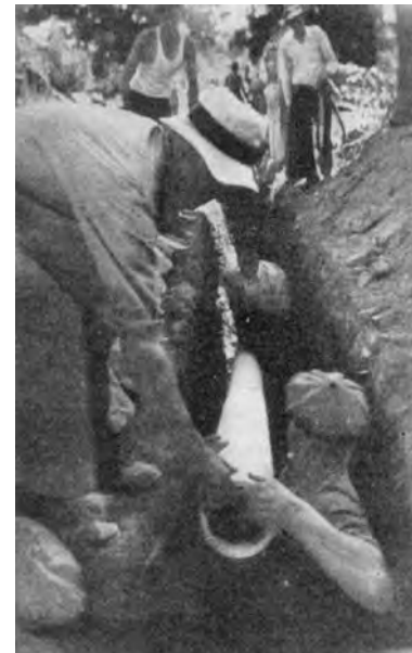
1937 Asbestos cement transite pipe laying, Note ease of handling.
