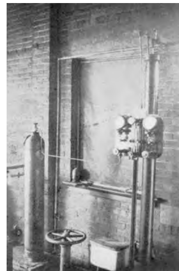
1916 Wakefield MA gas chlorinator – 1st in Massachusetts
