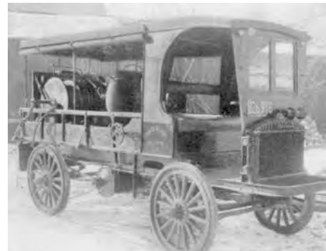
1920 pipe thawing truck using a portable generator for electric current, Dedham MA
