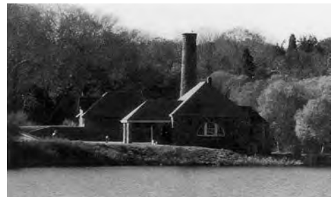
Oak Bluffs Pump Station, Martha's Vinyard MA
