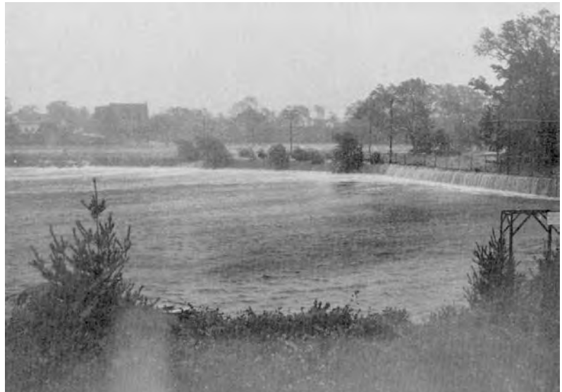
1954 Tidal surge ocean water pouring into Kickemuit Res., Bristol RI
