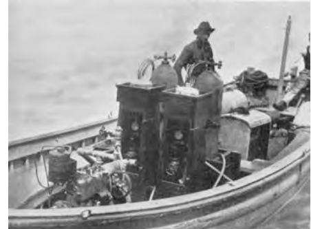
1924 Chlorine gas application to reservoir
