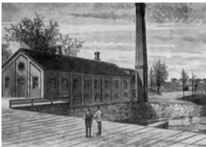
Pawtucket Pump Station, Pawtucket RI
