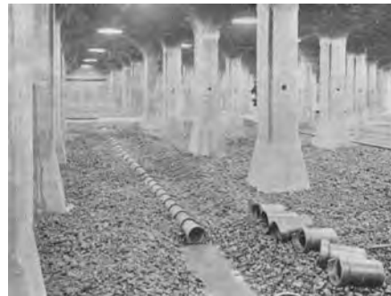
1918 Providence RI slow sand filter interior
