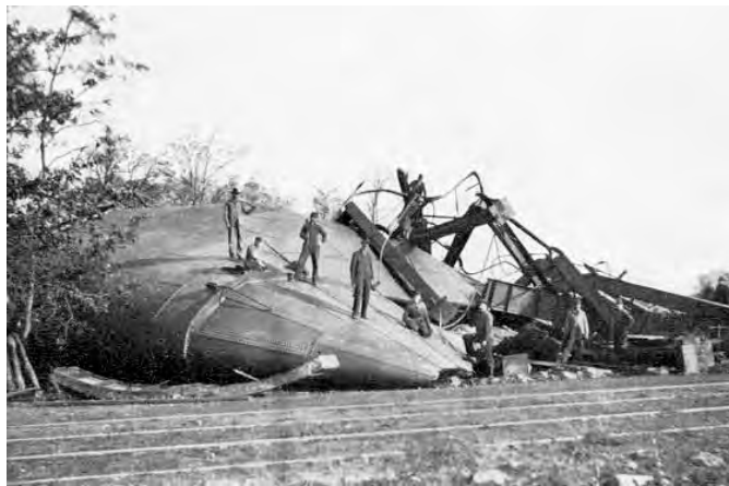
1901 Fairhaven MA Tank after the failure
