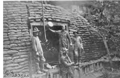
“Hardened” pump station at St. Jacques
