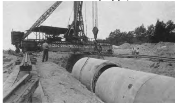
1946 laying Hultman Aq 138" RCP
