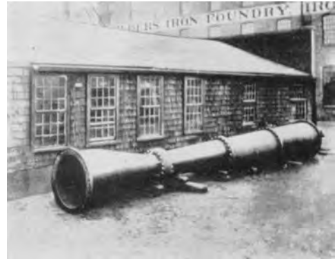
BIF's first venturi tube
