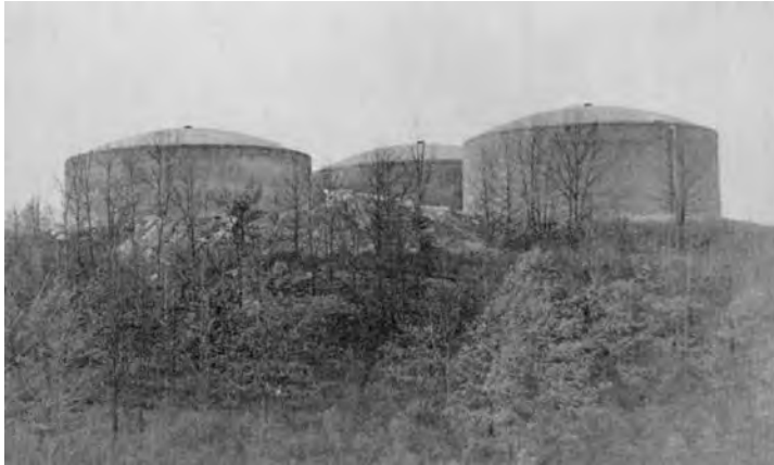
New London CT prestressed concrete tanks, failure occurred at pipe manifold in center
