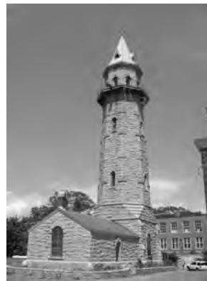
1884 Fall River MA Standpipe, contains two 42" riser pipes
