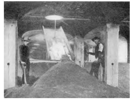
1918 Providence RI slow sand filter interior
