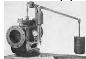
1906 Counterweighted pressure regulating valve
