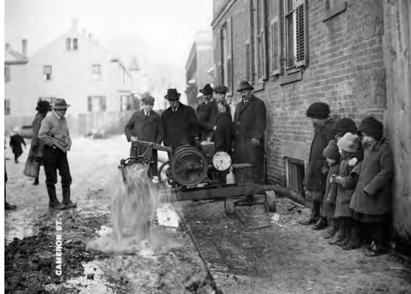
1916 Pumping out a basement after a 48” pipe break in Boston MA
