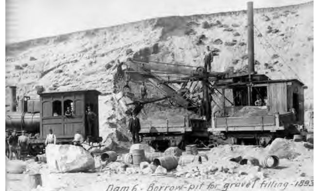
Dam excavation with a steam shovel
