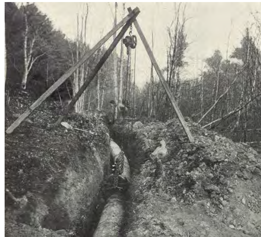
1916 14” wood stave pipe and valve, Pembroke NH
