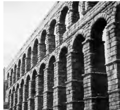
Roman Aqueduct bridge – the classic solution to moving water long distances across valleys
