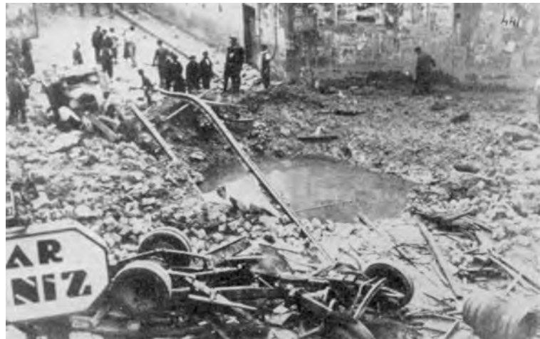
WW II Bomb crater in England, water leaking from broken main
