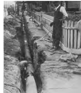
1927 welding steel pipe
