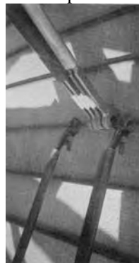
1942 turnbuckle prestressing system
