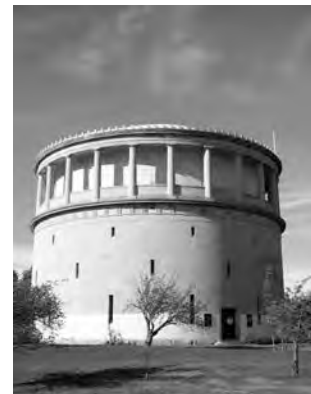
1921 Park Circle Standpipe, Arlington MA
