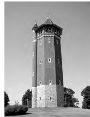
1895 Lawrence Tower, MA, AWWA Historical Landmark
