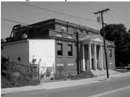
1938 Rapid sand plant
