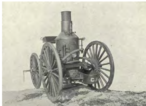
1904 Mobile boiler for pipe thawing, Manchester NH
