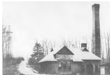
North Easton Pump Station, MA, AWWA Historical Landmark
