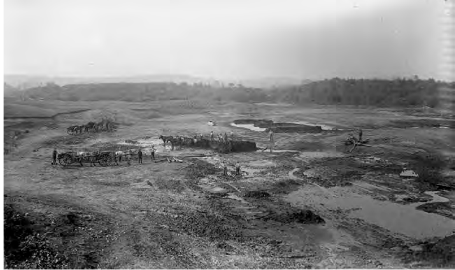
1898 Stripping the bottom of Boston's Sudbury Reservoir with horse drawn scrapers
