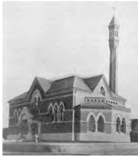
Hope Pump Station, Providence RI
