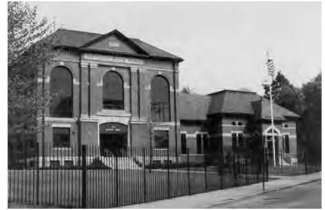
Branch Street Pump Station, Pawtucket RI, AWWA Historical Landmark
