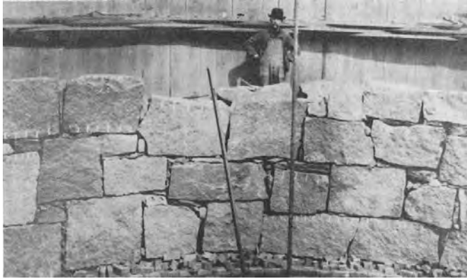
Inside Attleboro's dug well
