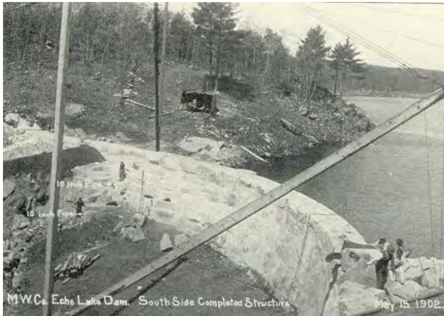
1902 Milford MA Masonry Dam
