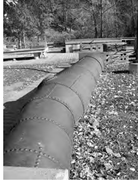
Example of wrought iron pipe, New Haven CT Water Interpretive Center
