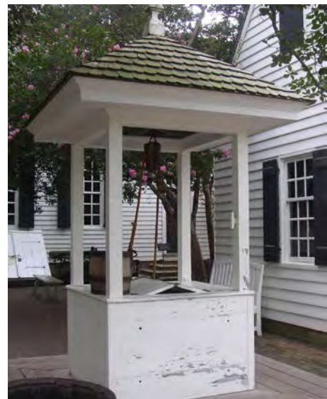
Typical household dug well from 1700's with bucket on rope pulley
