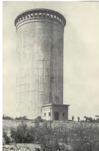
1906 Attleboro Standpipe completed
