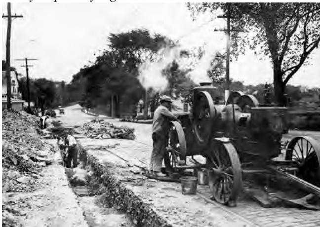
Breaking rock the old way, with a pneumatic jack hammer
