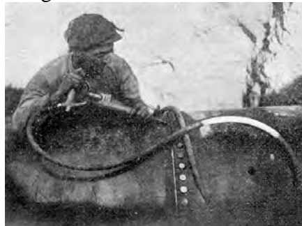
1924 caulking lockbar pipe
