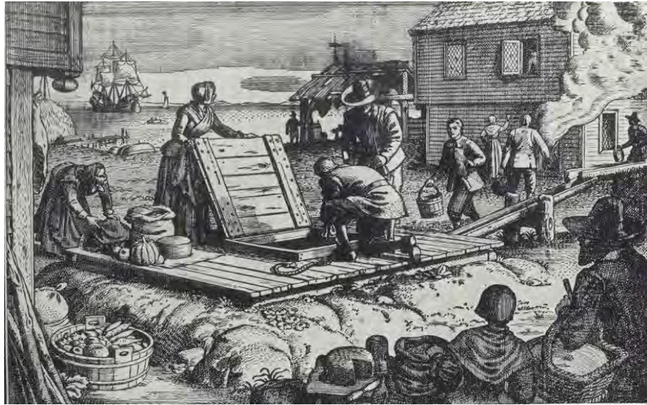
The "Conduit", Boston's 1652 supply, the first Water Works in the U.S.
