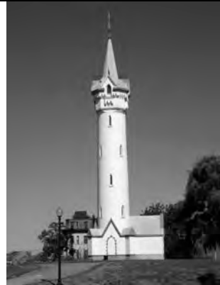
1870 Fort Hill Standpipe, Roxbury MA
