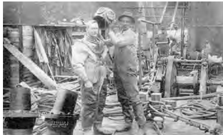
1895 Burlington VT diver, placing the intake pipe further in the lake.
