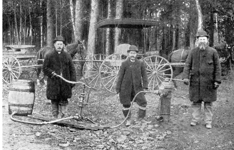
1896 – Some of New England's finest working on pipe pressure testing using a hand pump
