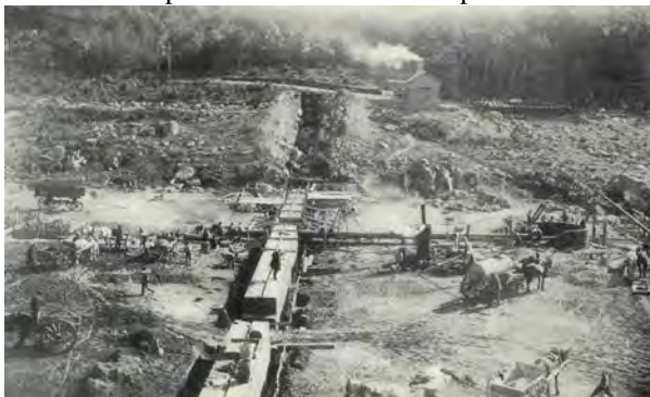
1905 Construction of Gloucester MA dam corewall
