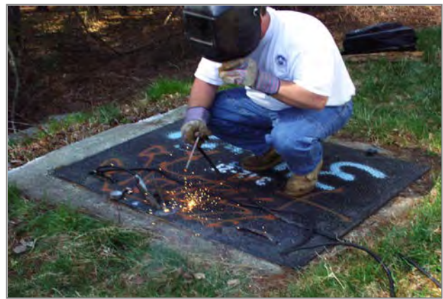
Post 9/11 Welding hatch covers
