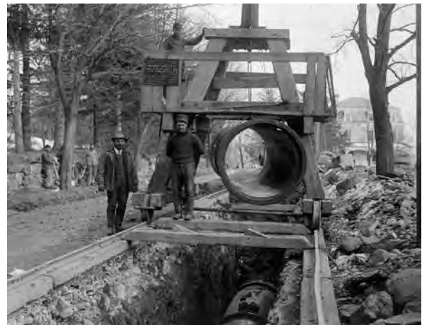
Early trenching machine
