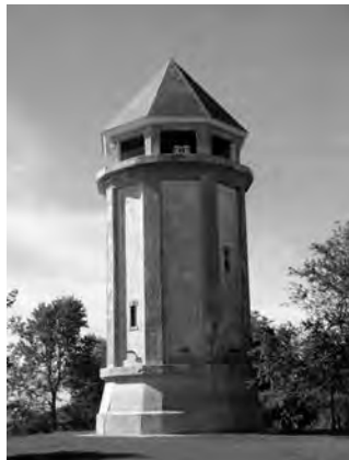
1903 Fort Revere Water Tower, Hull MA, was the first reinforced concrete standpipe in the US, AWWA Historical Landmark
