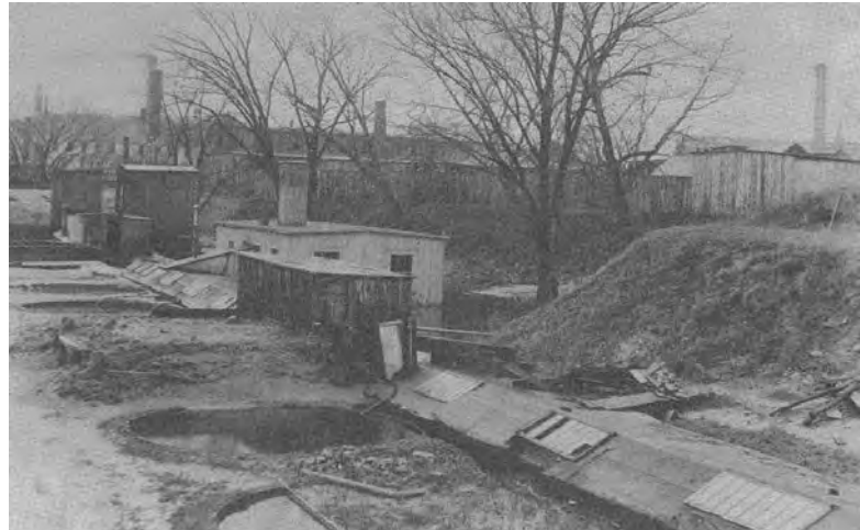
Original Lawrence Experiment Station buildings
