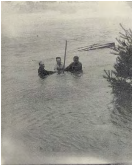
1954 Hurricane – Bristol RI staff closing a valve during the storm
