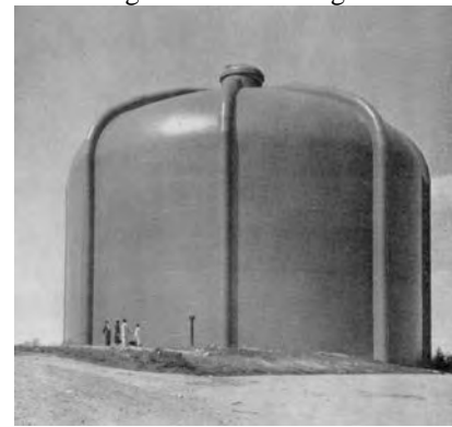
1961 Bellevue Tank, West Roxbury MA featuring ribs for the access ladders
