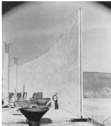
1959 Precast wall sections with integral waterproof core
