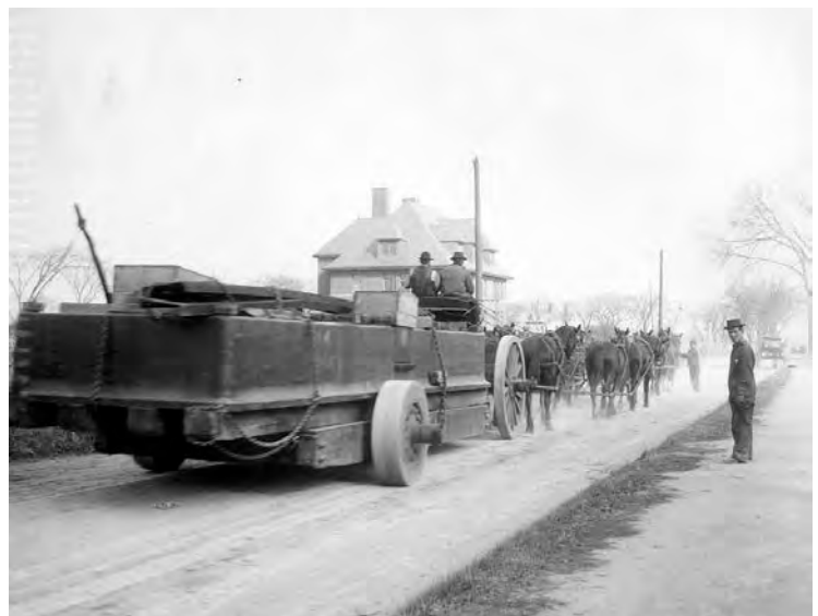
Moving a 50,000 lb steam pump base plate from railcar to site
