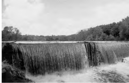
1860 Lake Whitney Dam serving New Haven CT
