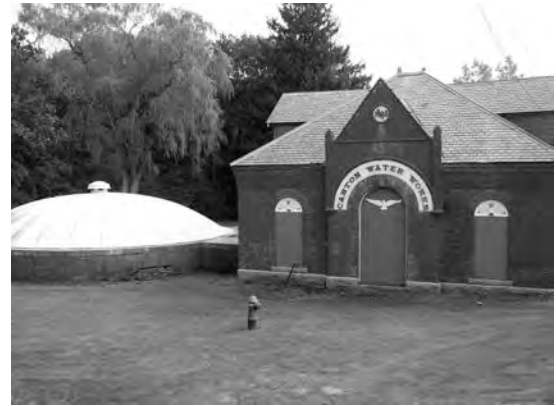
1887 Canton MA pump station adjacent to covered dug well
