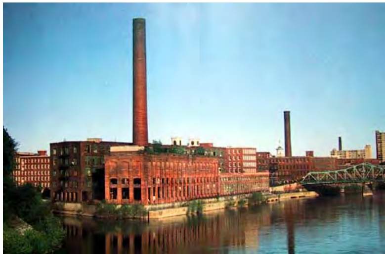
Lowell Mills on the Merrimack River, supplied from a canal network
