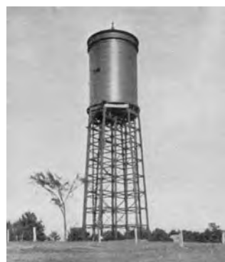
1905 East Providence RI Cast iron tank
