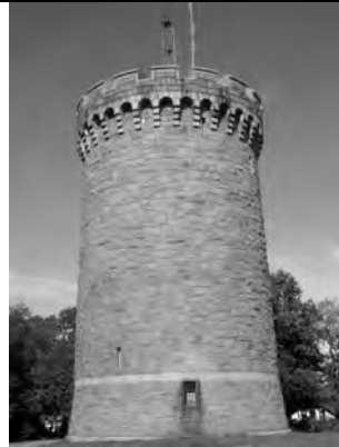
1902 Forbes Hill Standpipe, Quincy MA
