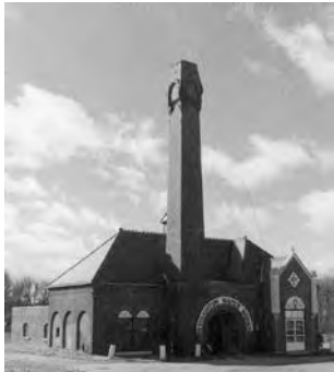
Stoughton Pump Station, MA
