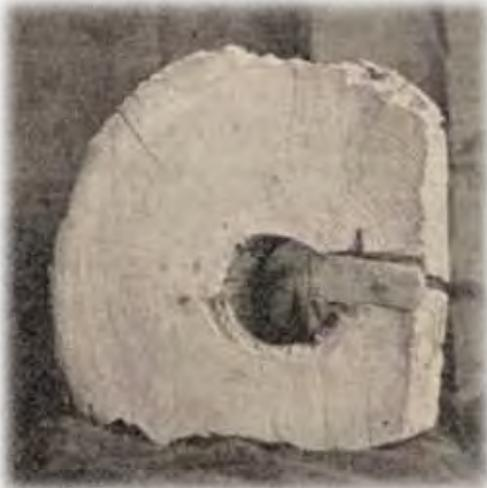
*Service connections were usually lead pipes but fire fighting access was drilled and refilled with wooden plugs (fireplugs)*
