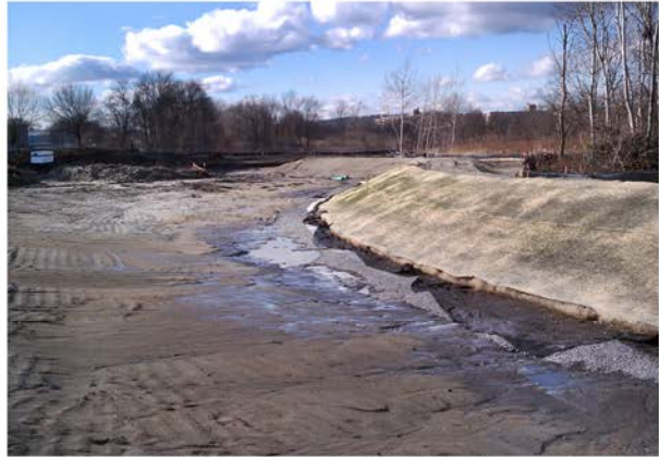
Perimeter Berm at Future Wetland Basin
