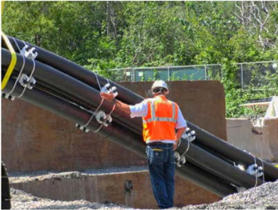
Launching Electric Bundle into Pit
