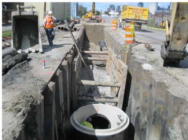
42" sewer and 16" water main installation on West First Street
