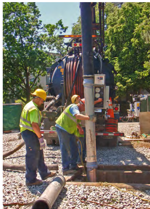
Contractor removing sediment from CSO Outfall MWR010
