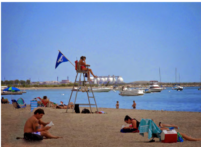
Carson Beach, with its long distance view of the Deer Island Wastewater Treatment Plant
