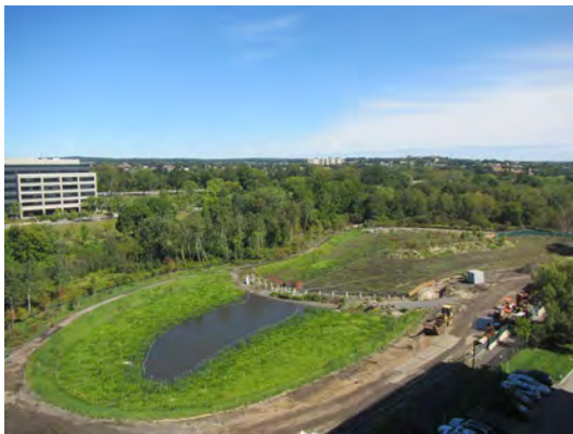
Main Wetland Basin, West to East, November 2012
