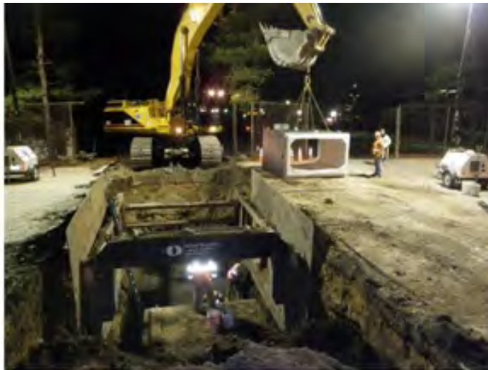
Nighttime Construction of Stormwater Box Conduit on Upper Wheeler Street, February 2012
