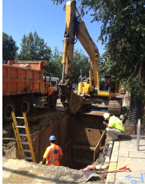
Trenching along Beacon Street, Brookline, August 2012
