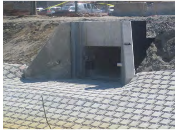
Storm Drain Outfall to Forebay, March 2012
