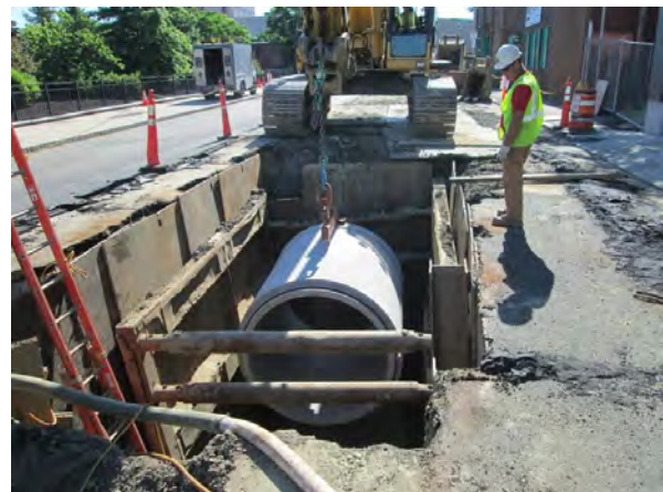
Storm Drain Installation on E. First St. (Contract 3B)
