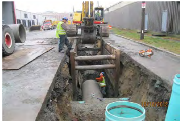
Installation of 36-inch Storm Drain on E St. (Contract 4)
