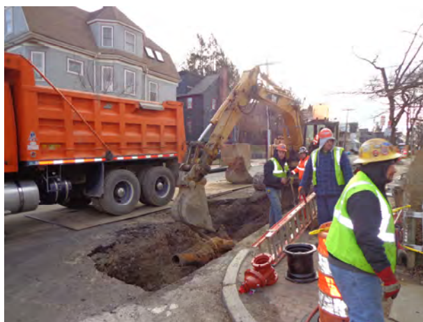
Water Main Relocation Work Ahead of Sewer and Storm Drain Installation on Lexington Avenue at Huron Avenue
