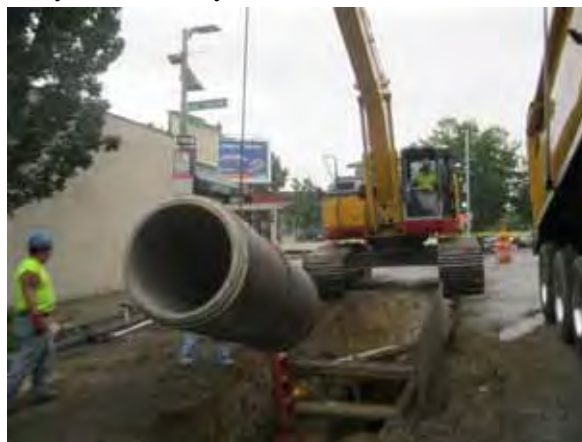
Installation of 30-inch drain on I Street Reserved Channel Contract 4
