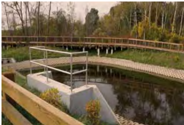
Stormwater outfall and basin "Forebay"
