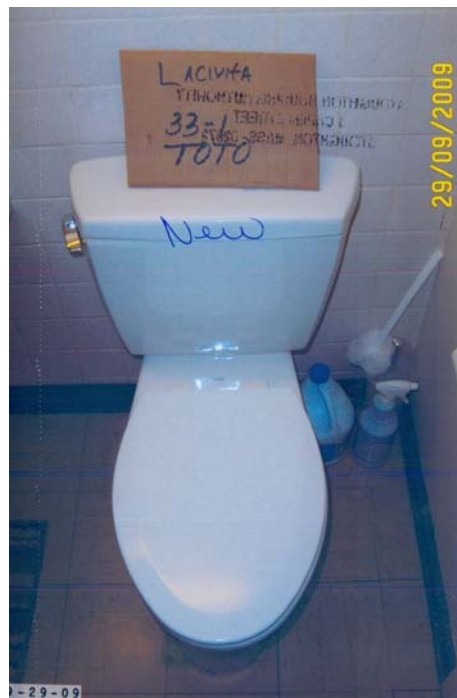
Figure 2 - Sample Low-Flow Toilet After Retrofit
