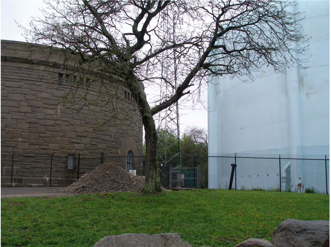
Bellevue Storage Tanks
