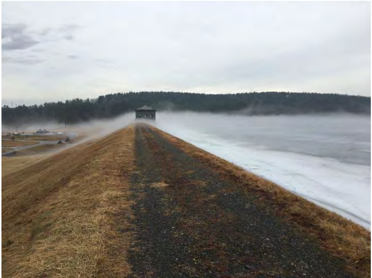
Fog creeping in over Sudbury Dam
