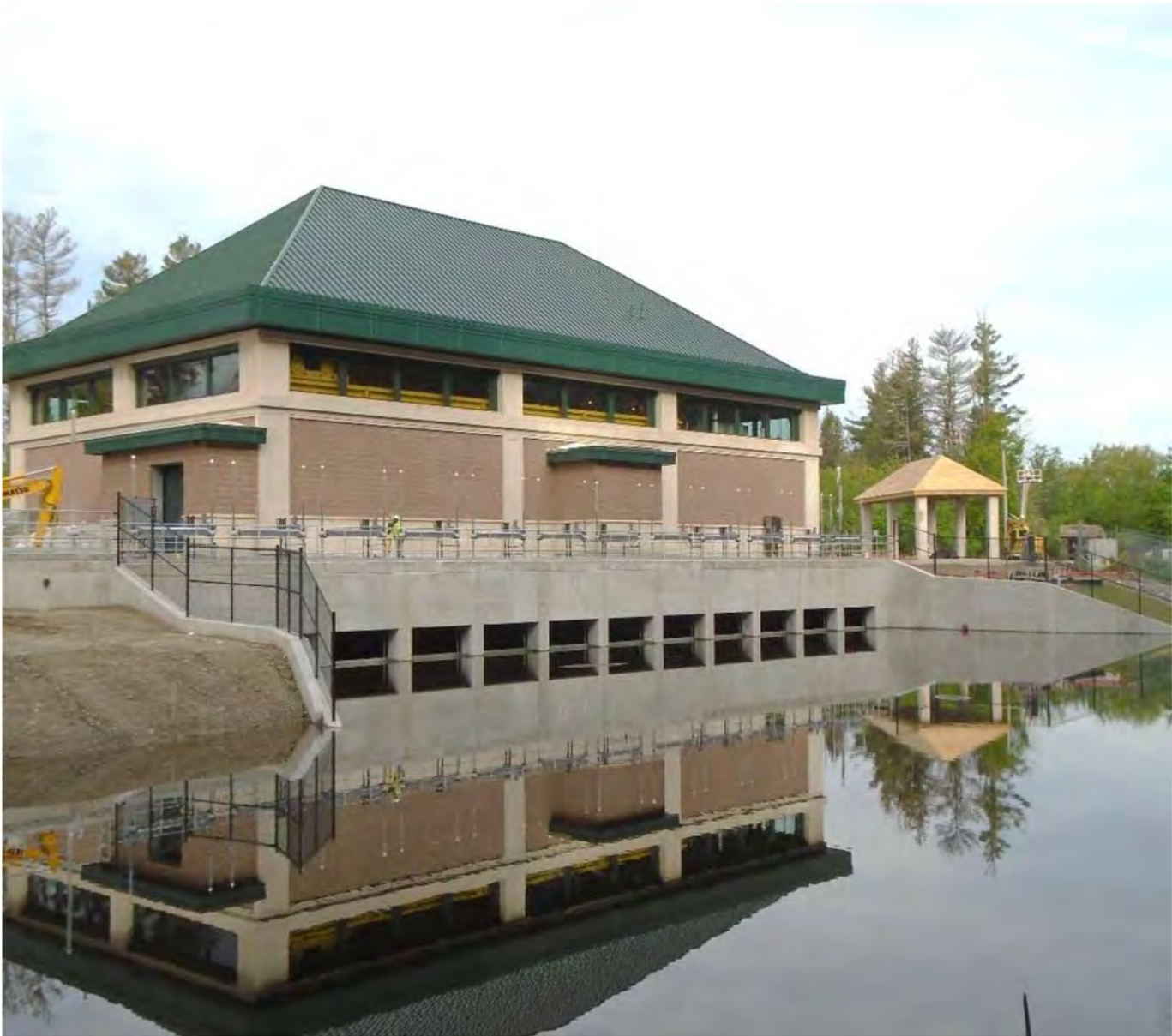
Wachusett Aqueduct Water Pump Station Forebay
