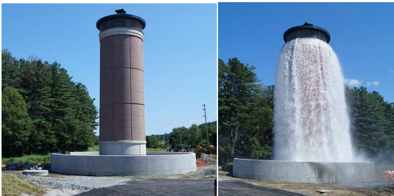
Wachusett Aqueduct Pump Station Surge Structure
