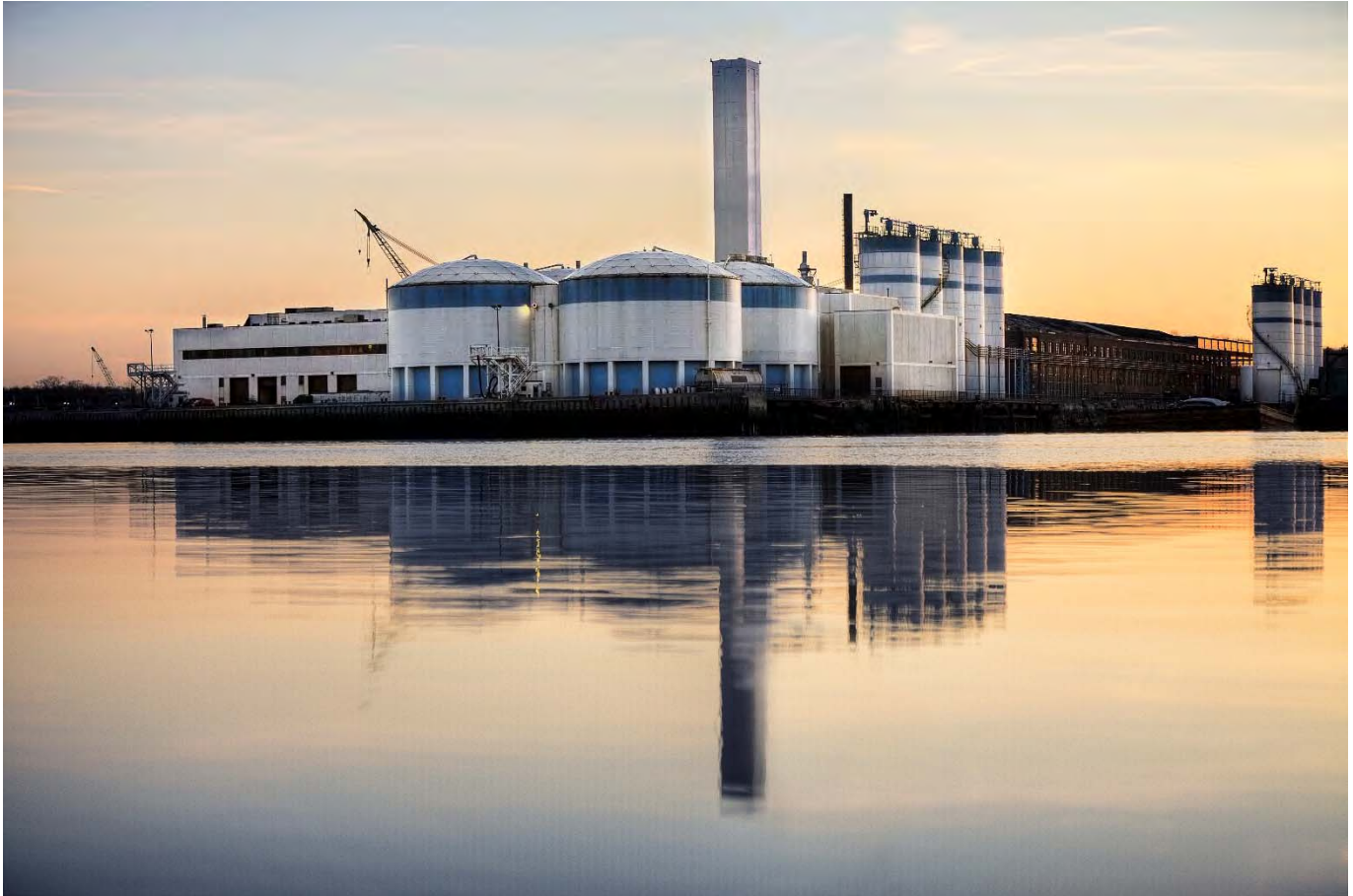
MWRA Sludge Pelletizing Facility
