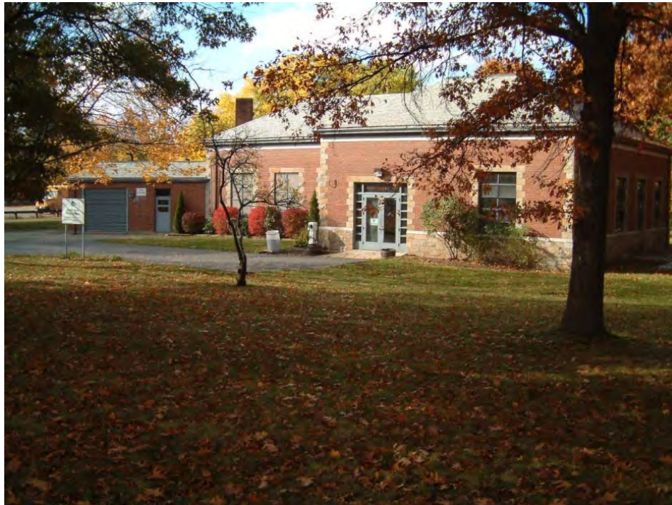
Alewife Brook Wastewater Pump Station
