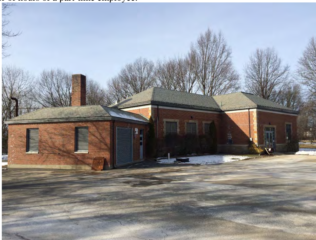
Alewife Brook Wastewater Pump Station
