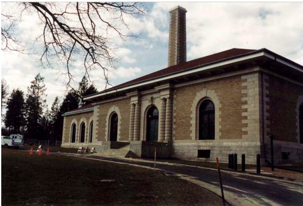
Gillis Water Pump Station
