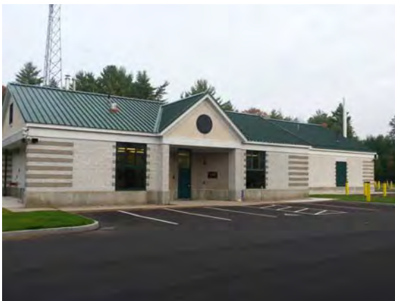
Brutsch Water Treatment Facility
