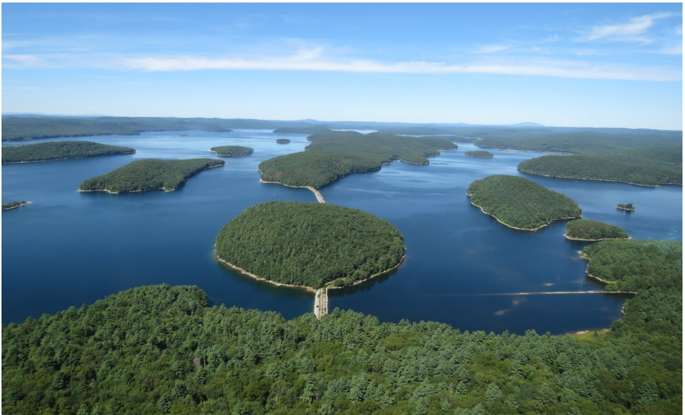
Baffle Dams Quabbin Reservoir
