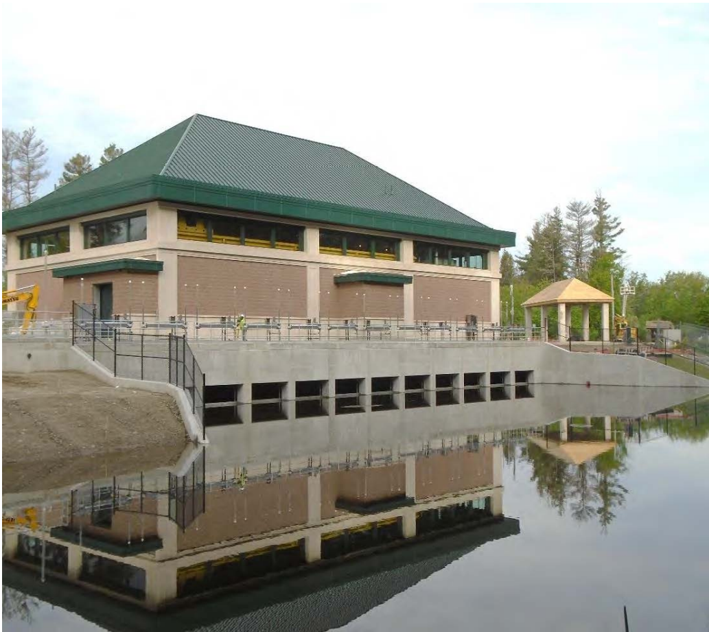
Wachusett Aqueduct Water Pump Station Forebay
