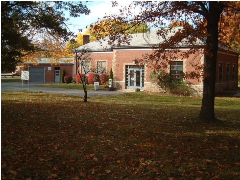
Alewife Brook Wastewater Pump Station
