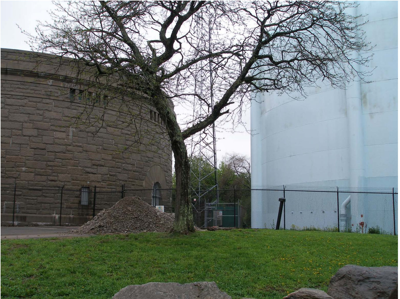
Bellevue Storage Tanks
