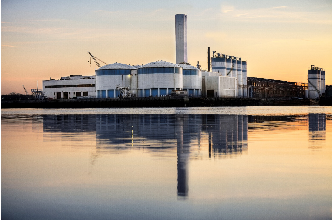
MWRA Sludge Pelletizing Facility
