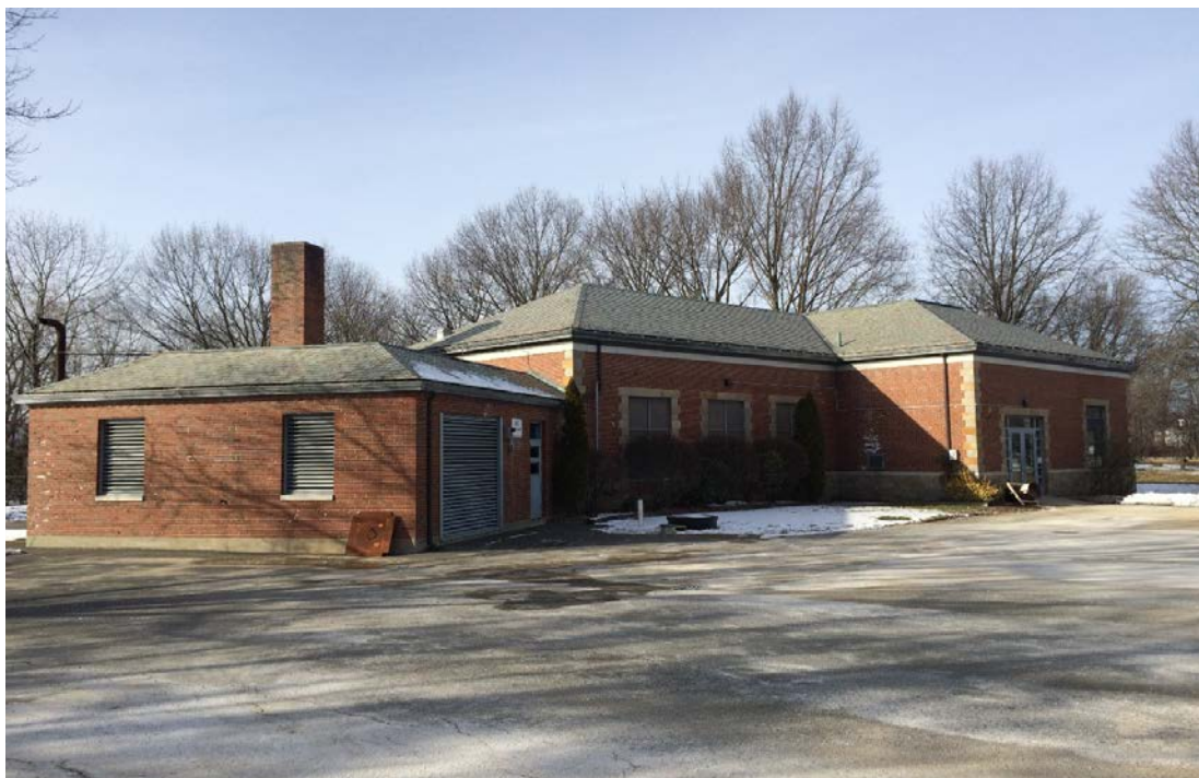
Alewife Brook Wastewater Pump Station
