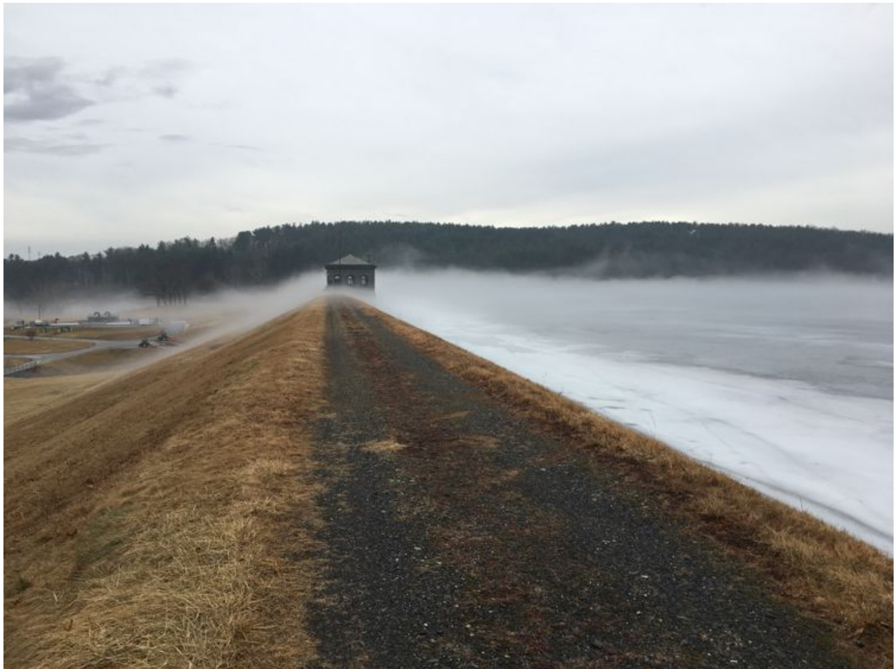
Fog creeping in over Sudbury Dam
