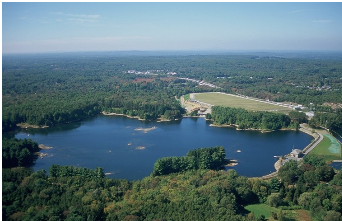
Norumbega Covered Storage Tank
