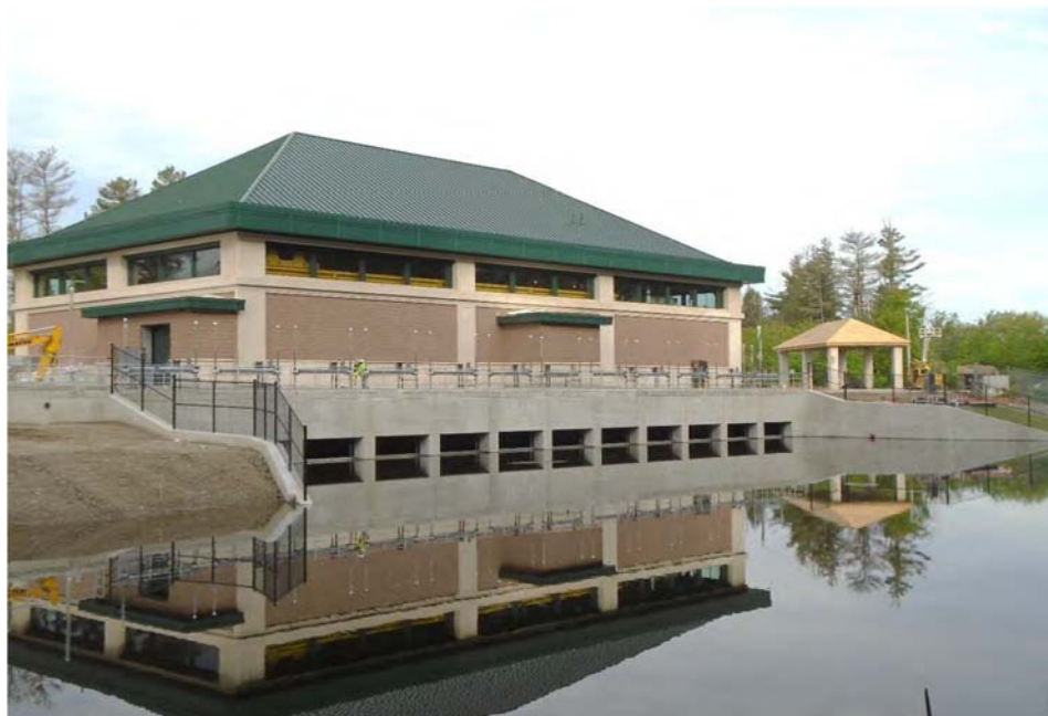
Wachusett Aqueduct Water Pump Station Forebay
