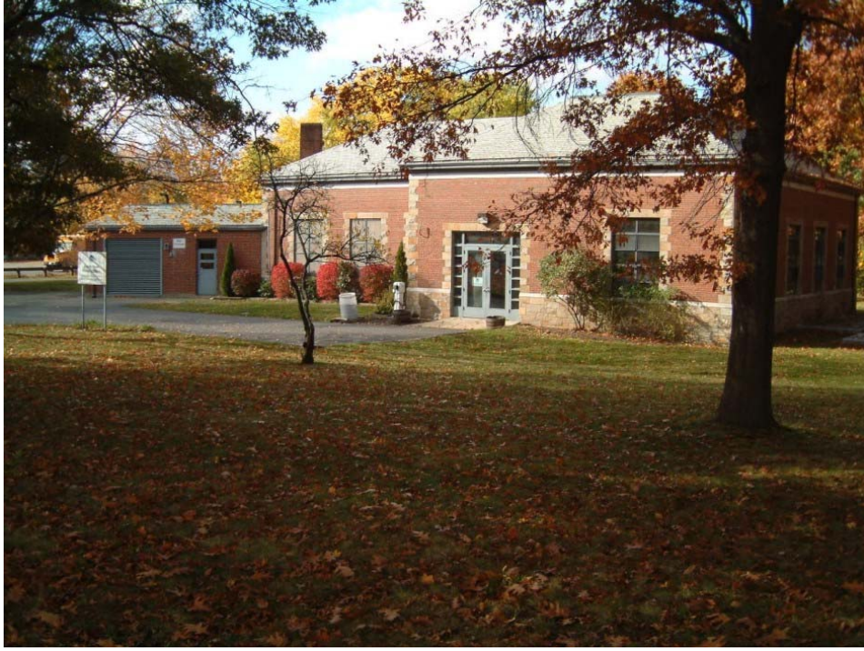
Alewife Brook Wastewater Pump Station
