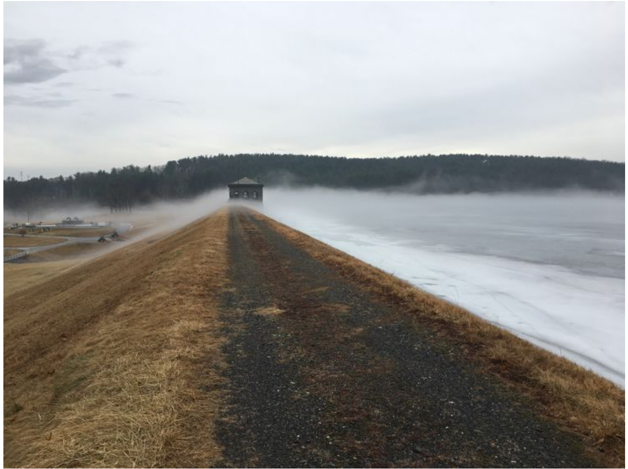
Fog creeping in over Sudbury Dam
