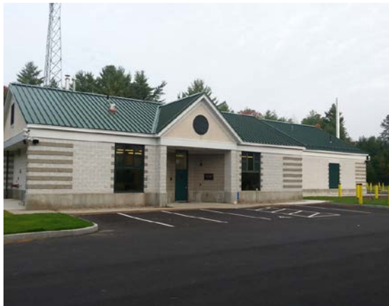
Brutsch Water Treatment Facility
