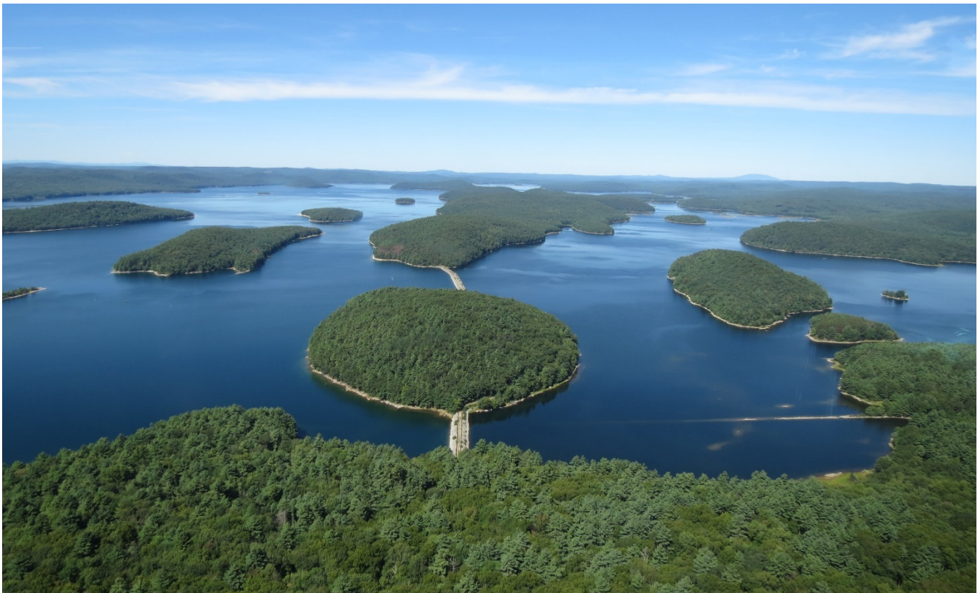
Baffle Dams Quabbin Reservoir
