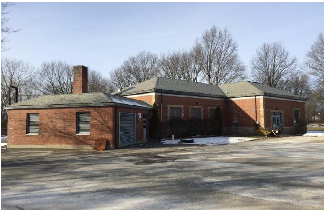
Alewife Brook Wastewater Pump Station
