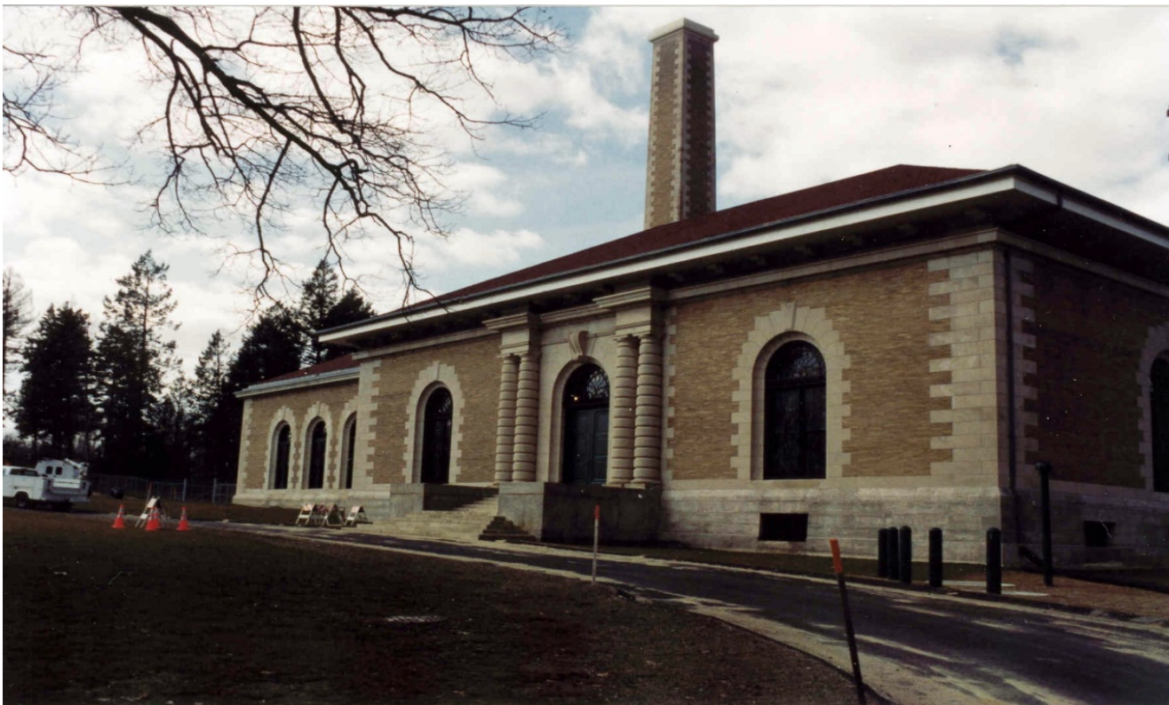
Gillis Water Pump Station
