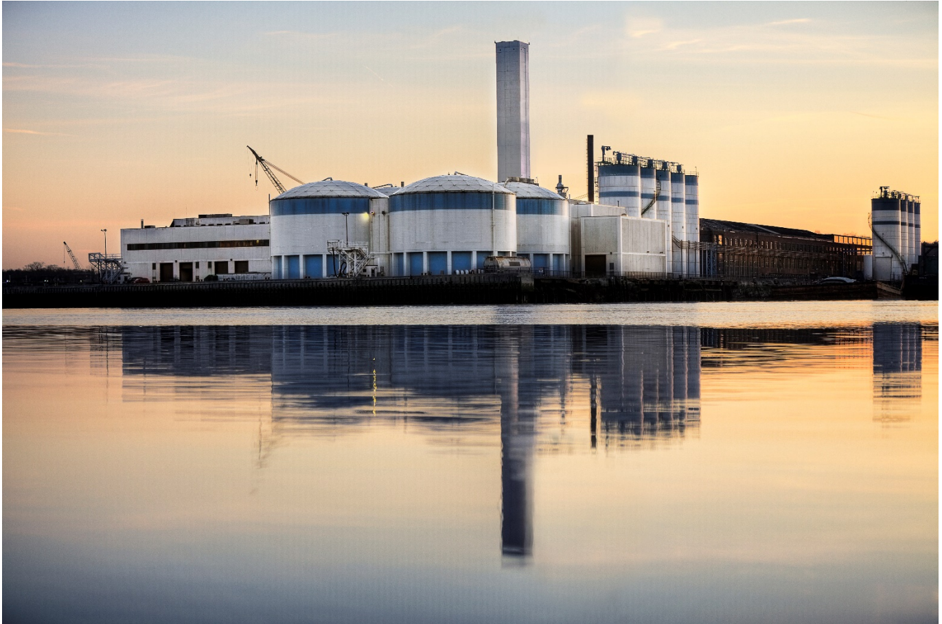
MWRA Sludge Pelletizing Facility
