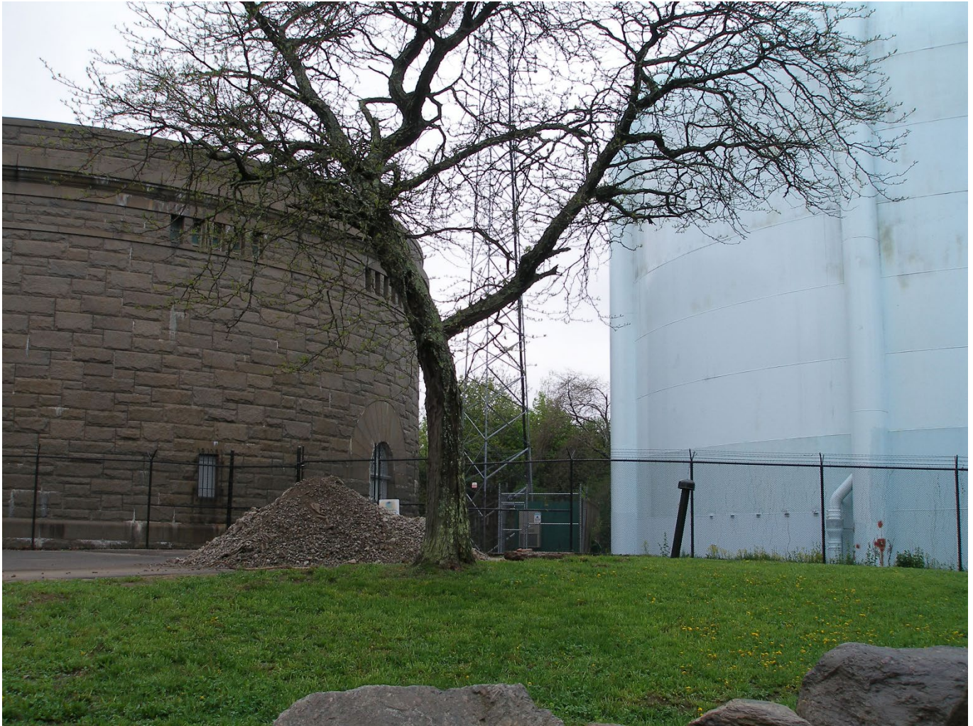
Bellevue Storage Tanks
