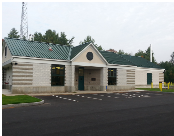
Brutsch Water Treatment Facility
