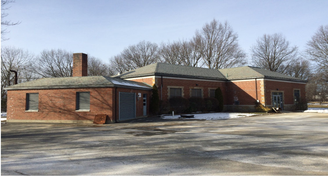
Alewife Brook Wastewater Pump Station
