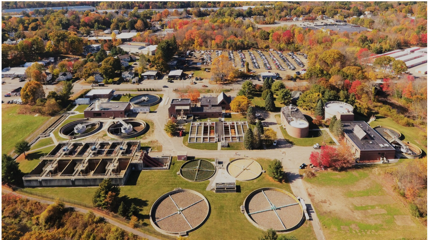
Clinton Wastewater Treatment Plant
