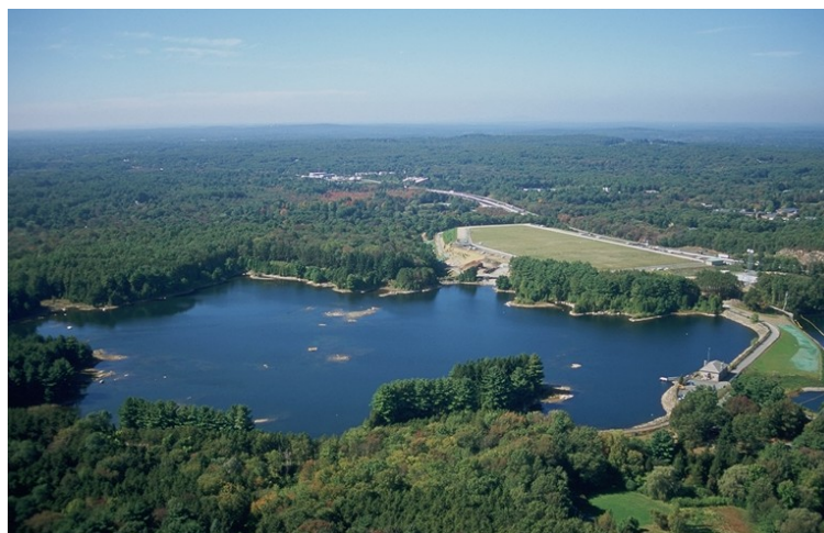
Norumbega Covered Storage Tank and Norumbega Open Reservoir (now a backup supply)
