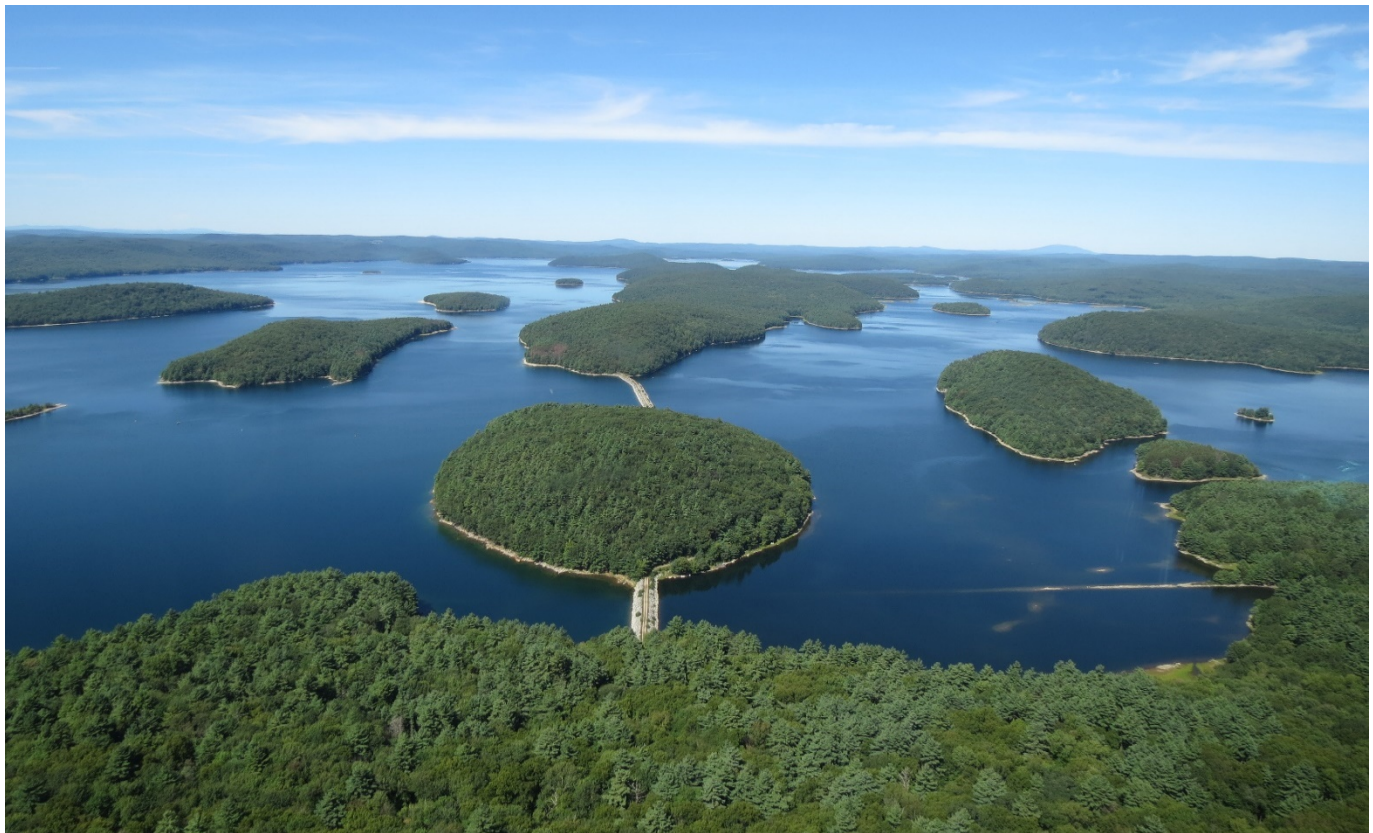
Baffle Dams Quabbin Reservoir
