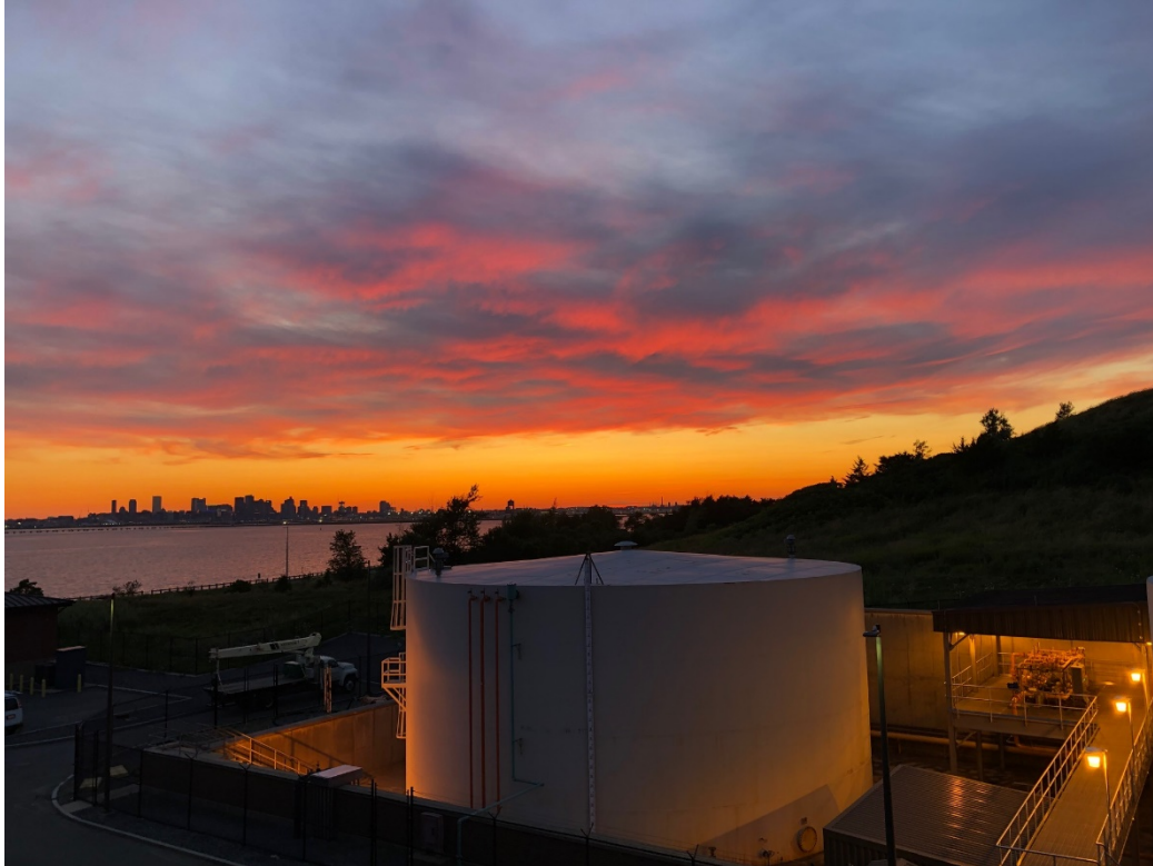
Deer Island Treatment Plant Thermal Power Plant
