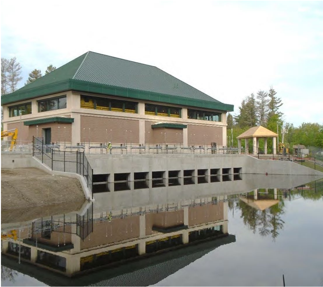
Wachusett Aqueduct Water Pump Station Forebay
