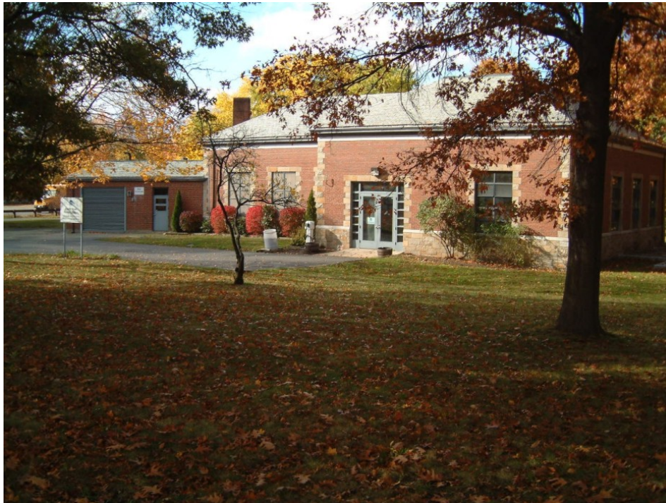
Alewife Brook Wastewater Pump Station
