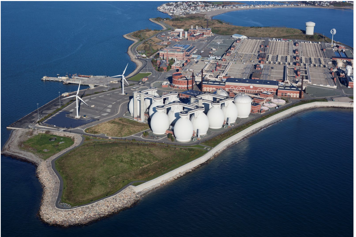
Deer Island Wastewater Treatment Plan
