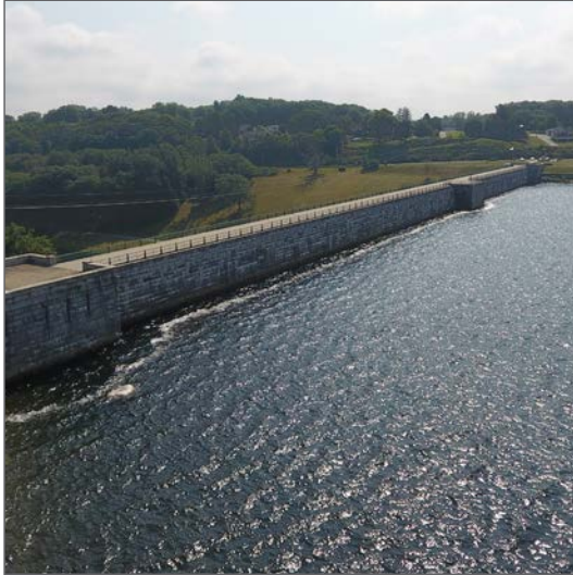
Wachusett Dam, Clinton
