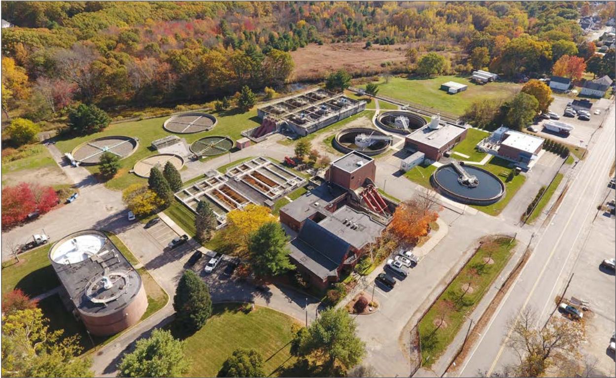
Clinton Wastewater Treatment Plant
