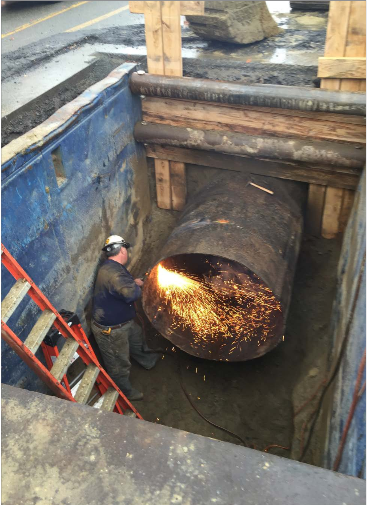
WASM3, Cutting 56" lock bar steel rivet pipe in Arlington
