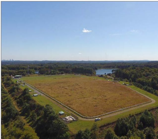
Norumbega Covered Storage Facility in Weston
