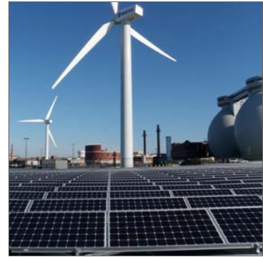
Wind turbines and solar panels at the Deer Island Wastewater Treatment Plant
