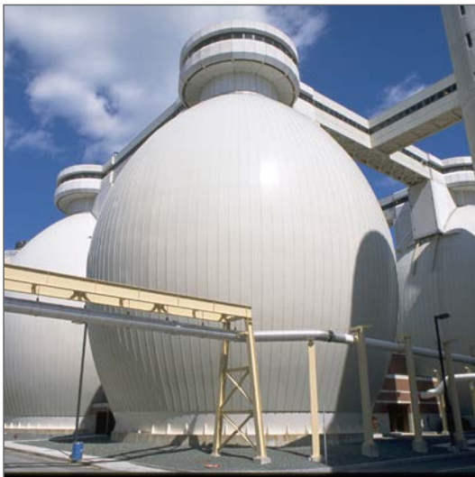
Digesters at Deer Island Treatment Plant
