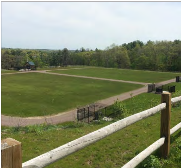
Spot Pond Covered Storage
