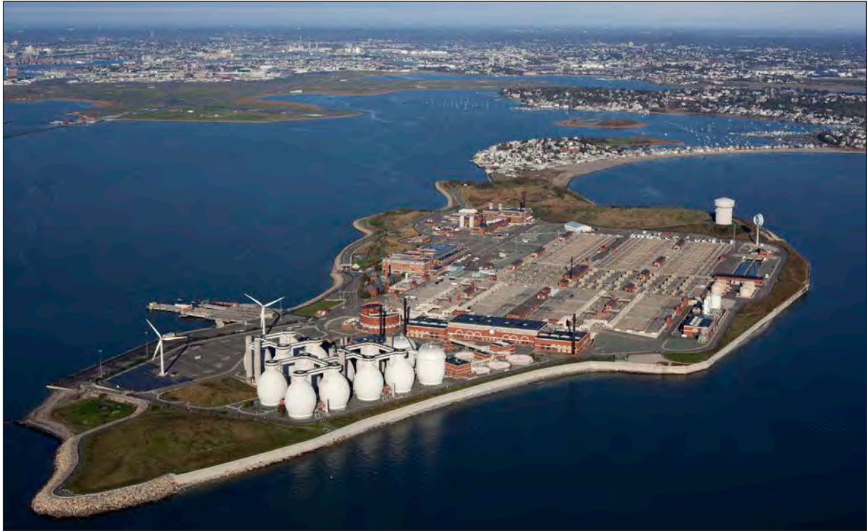
Deer Island Wastewater Treatment Plant
