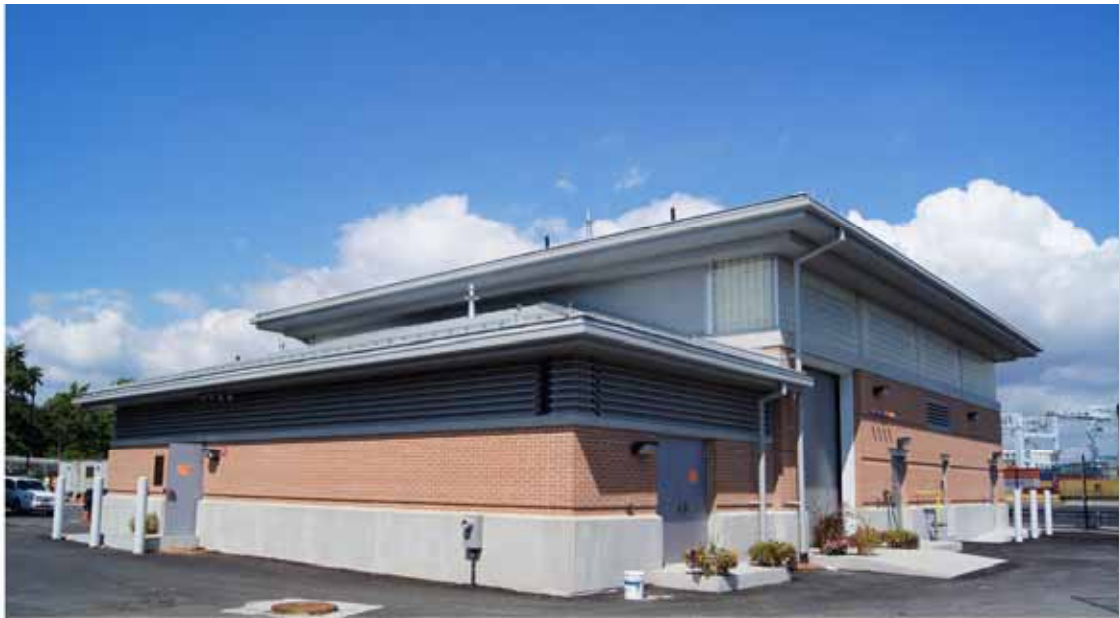
North Dorchester Bay CSO Storage Tunnel Dewatering Pump Station, Conley Terminal, South Boston
