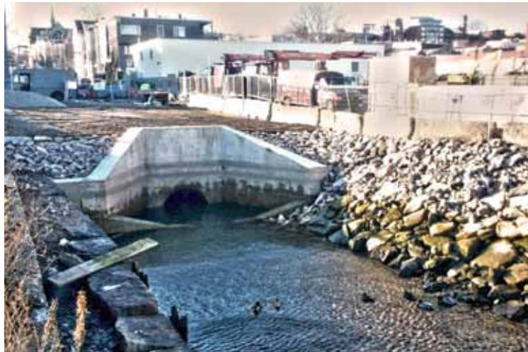
Completed Rehabilitation of Outfall BOS078
