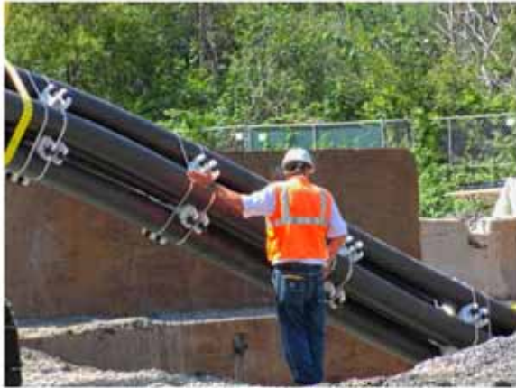
Launching Electric Bundle into Pit
