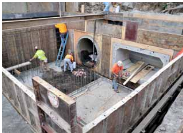
Stormwater Diversion Structure
