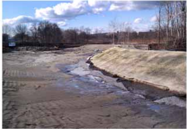
Perimeter Berm at Future Wetland Basin
