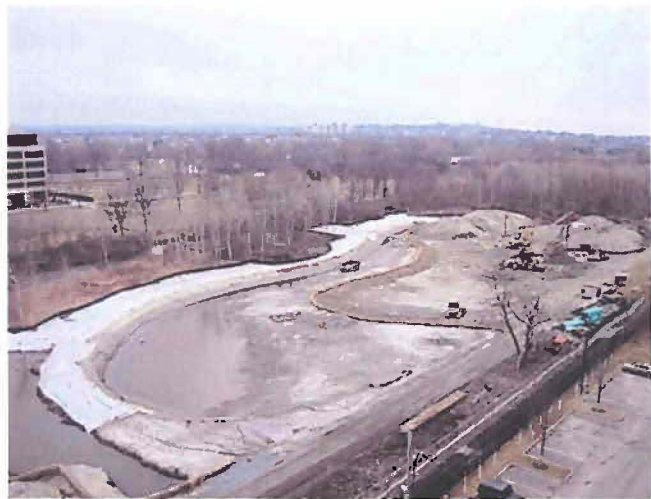
Fig. 2 - Stormwater Wetland Basin Construction
