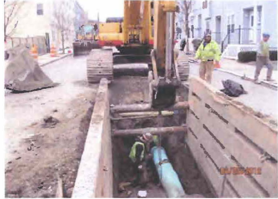
Figure 2: sewer installation on West Second Street
