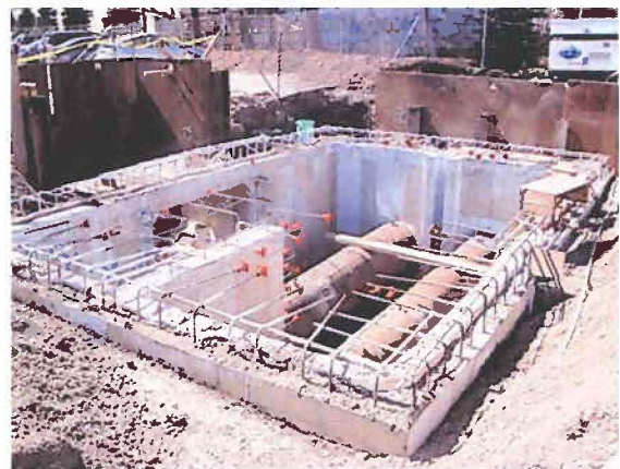
Fig. 1 - Crossing structure at MWRA interceptors behind 125 Cambridge Park Drive
