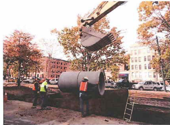
Figure 1 - Open Cut Trenching at Beacon St: Installation of Drain Line Segments
