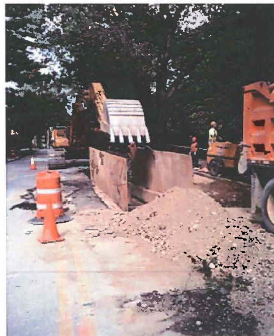
Figure 2 - Open Cut for Drain Line Installation at Carlton St
