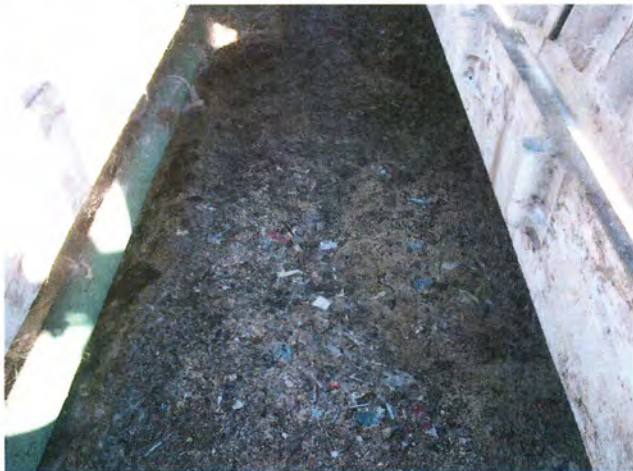
Scum and Rag Build-up in Secondary Influent Channel
