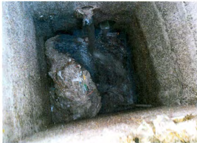
Rag Build-up in Gravity Thickener Scum and Overflow Well
