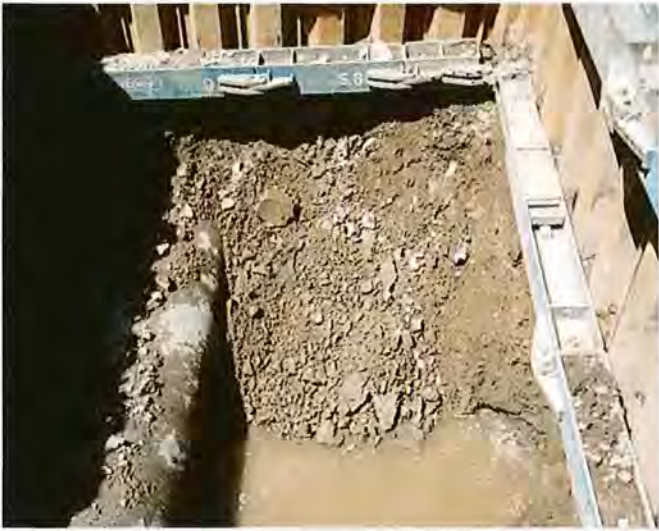
Ledge Croppings Inside Excavated Pit
