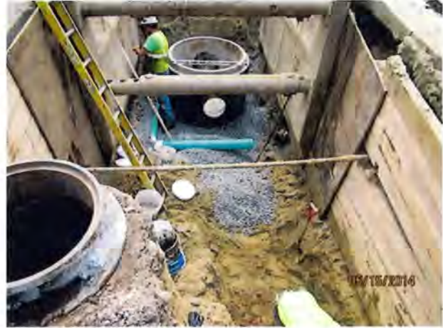
Drain Manhole 21 installation on Concord Avenue under Contract 9
