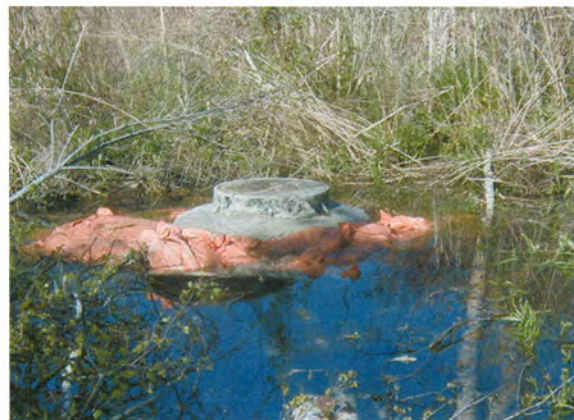
Sewer Manhole in Wetland - Raised and Sealed
