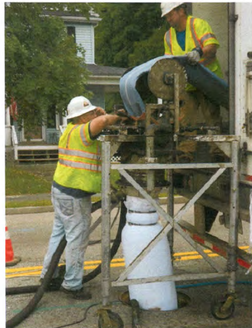
Installation of CIPP Pipe Liner
