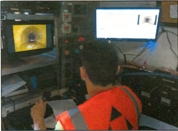
Sewer TV Inspection
