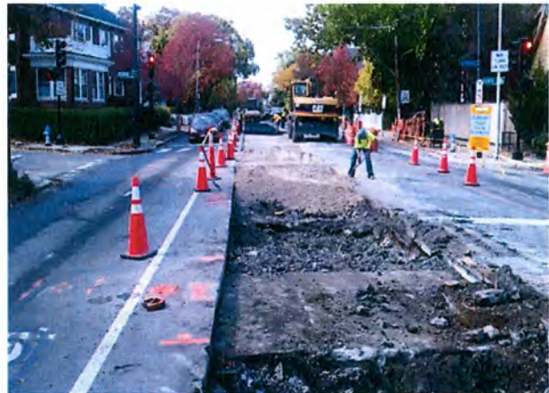
Removal of old rails on Huron Avenue, Contract 8B
