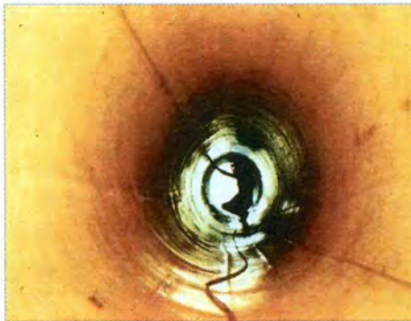
CIPP Pipe Liner
