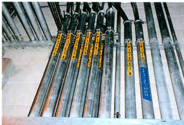
New Conduits in Electric Room
