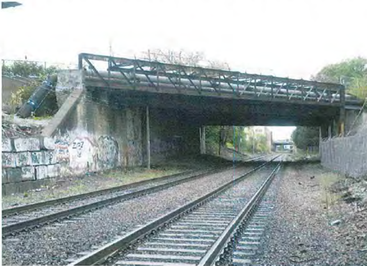
Pipe Bridge over Fitchburg Rail Line
