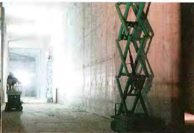
Concrete Finishing Work Inside the Tank
