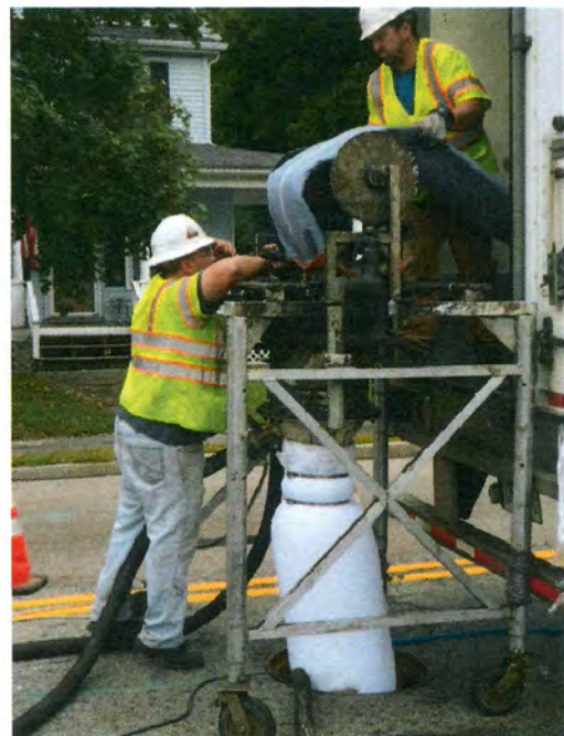
Installation of CIPP Pipe Liner
