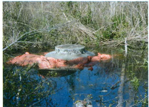
Sewer Manhole in Wetland - Raised and Sealed
