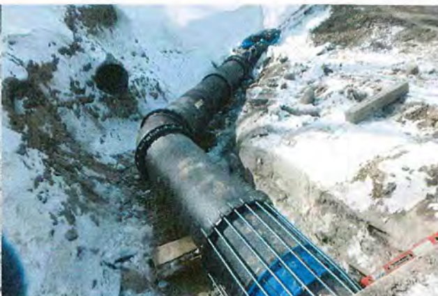
Yard Piping (Section 64 Tie-In), March 2015
