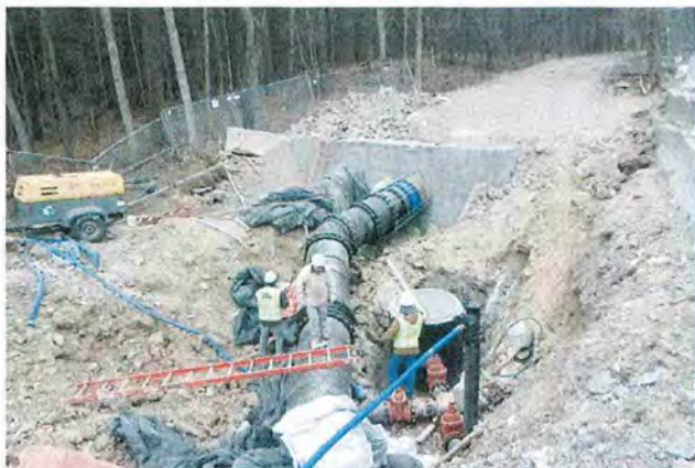
Yard Piping (Section 13 Tie-In), early January 2015
