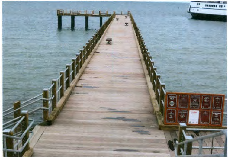
Similar Pier Installed In Oak Bluffs
