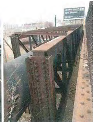
Only Utility Support Bridge to be Replaced
