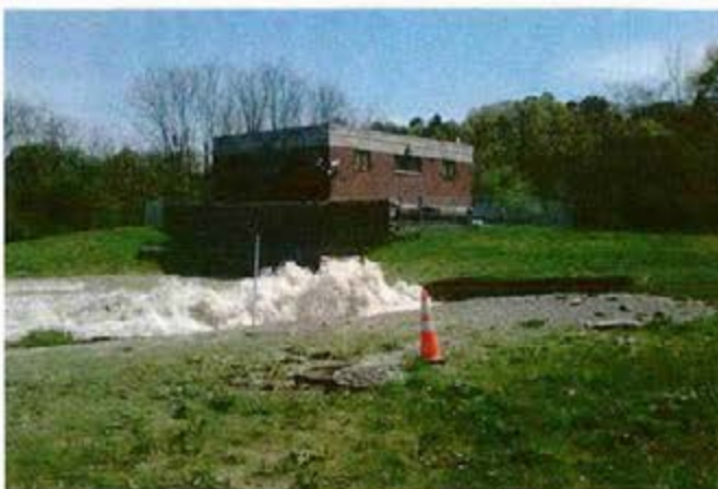
Shaft 5 Break. May 1, 2010
