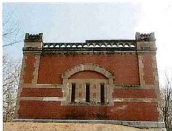
Current View East Building
