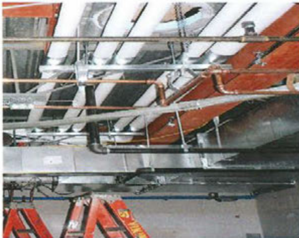
New HVAC Duct Work
