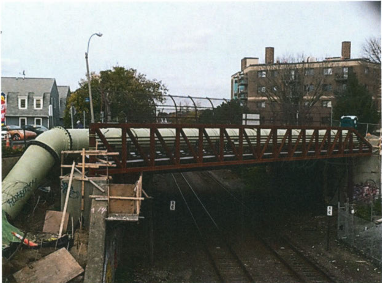
Figure 1. New 48-inch pipe and utility bridge.
