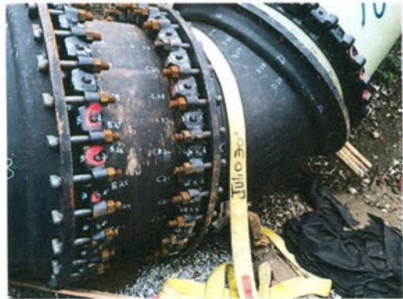
Figure 3. Horizontal and Vertical Bends on South side of bridge.
