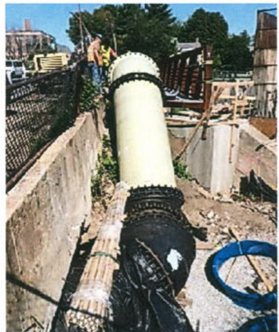
Figure 4. Vertical mechanical joints bends with Megalug restraints.
