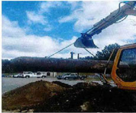
Propane Tank Removal
