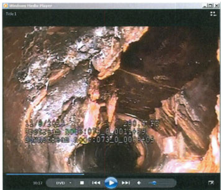
Reading Extension Sewer – Section 73
