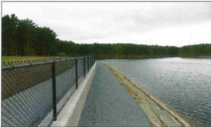
Figure 3. Weston Dam parapet wall
