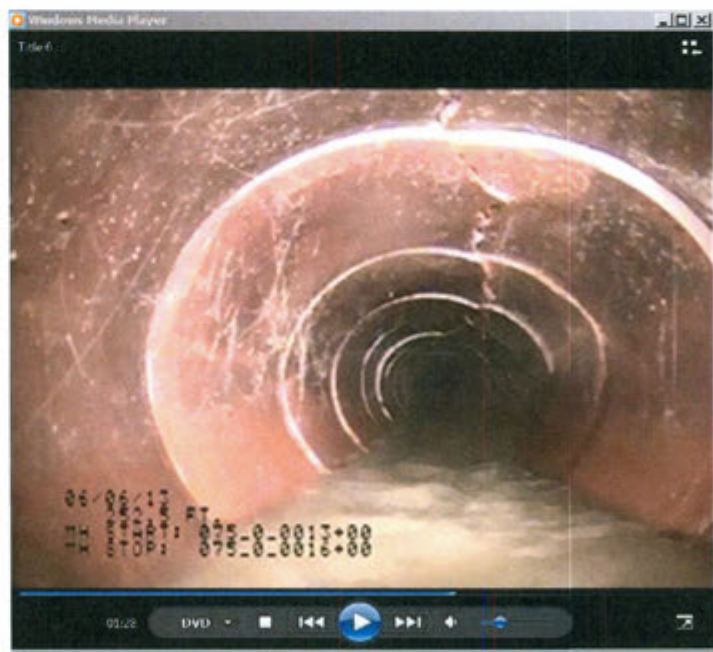
Reading Extension Sewer – Section 75
