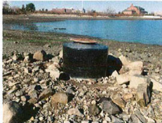
Sewer Manhole at Beach - Raised and Sealed
