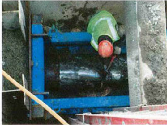
Sewer Replacement using Pipe Bursting
