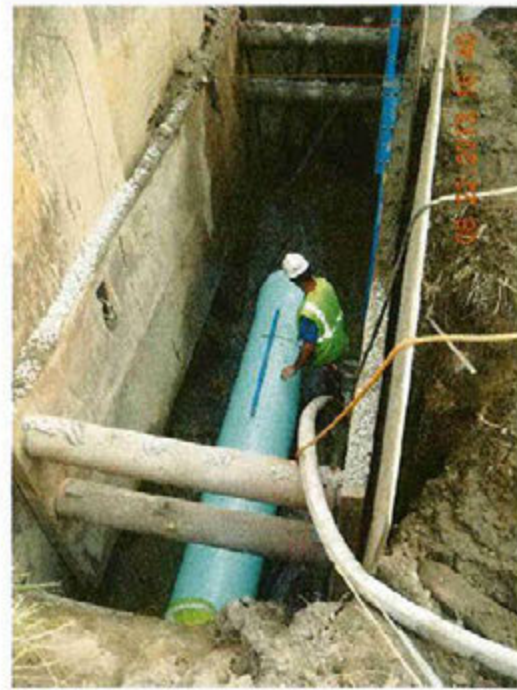
Installation of New PVC Sewer Pipe
