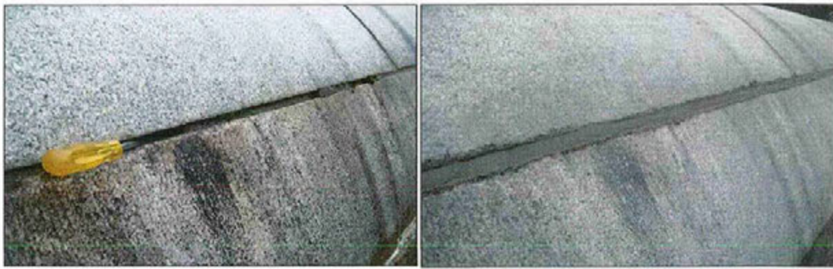
Figure 6. Quabbin spillway repairs (before L) and after (R)
