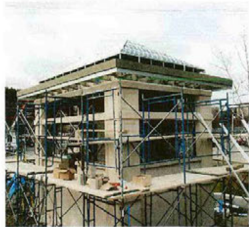
Guardhouse Progress Photo
