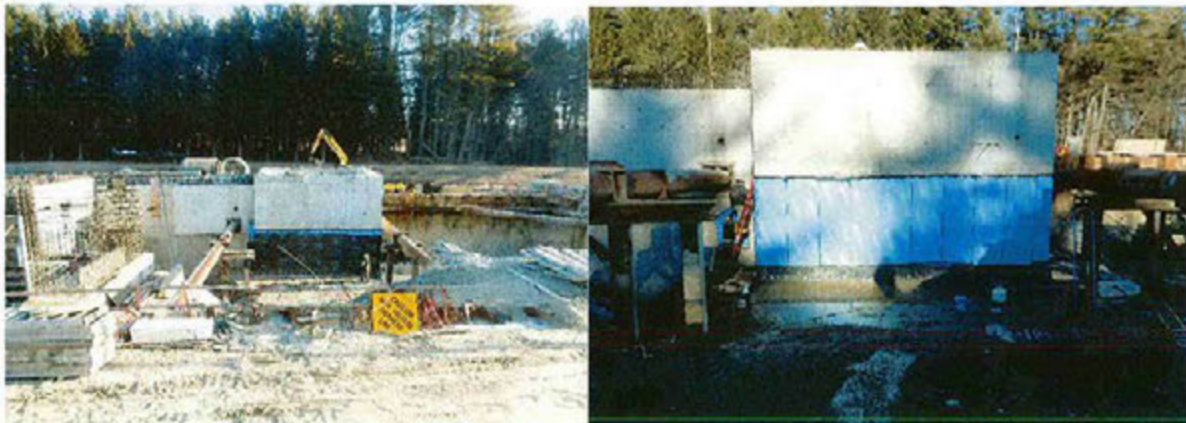
Waterproof membrane/protection board at South wall of the Butterfly Valve Vault
