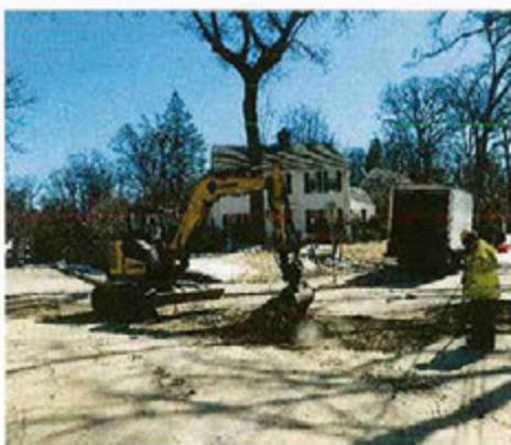
Installation of drain across Pine Ridge Road
