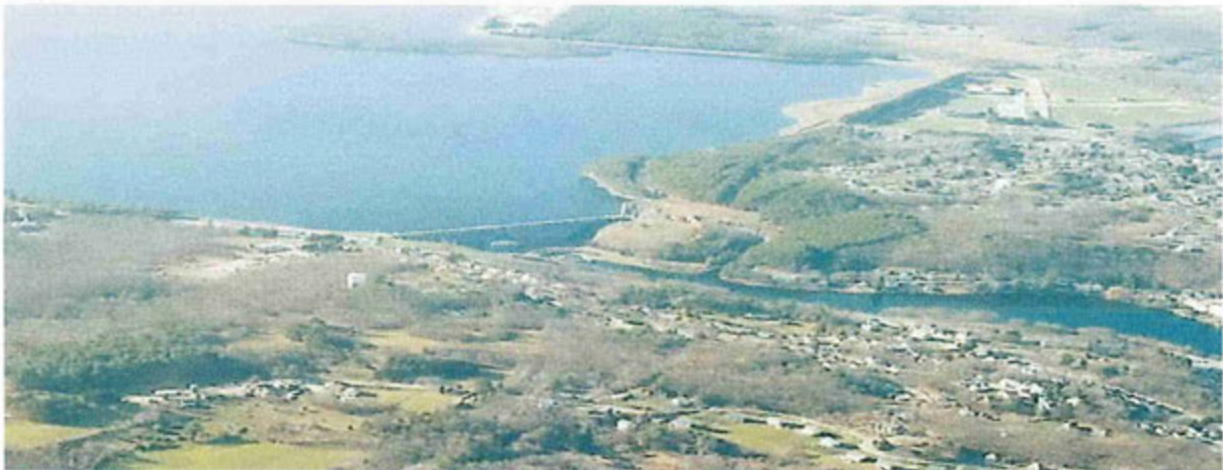
Wachusett Reservoir Dam and North Dike
