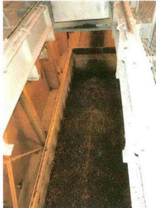
View of Grit Trailer from above Conveyor Drop Opening. Trailer Contains Approximately One Week's Accumulation
