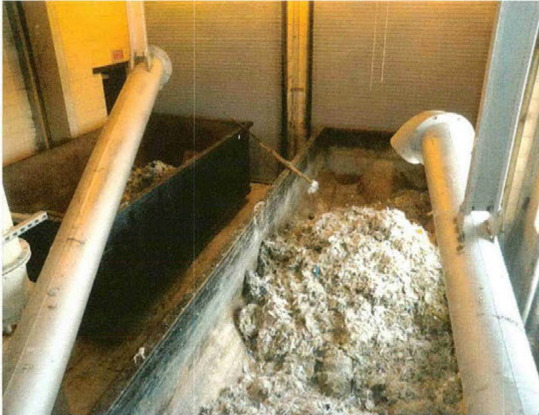
Partially Filled Roll-Off Containers Receiving Washed Screenings from the Removal System Conveyor (Not Shown) Discharge Piping at the Winthrop Terminal Facility
