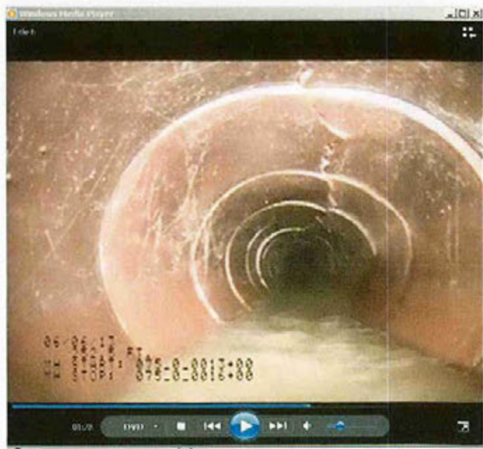
Reading Extension Sewer – Section 75
