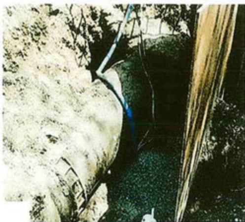
Section 80 – Test Pit of 48-inch Steel Pipe
