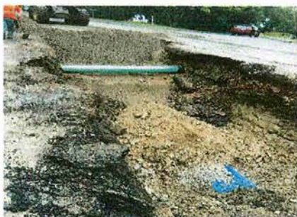
Drain removed and replaced
