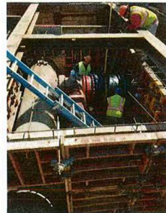
Solid Sleeve at the Section 77 Tap
