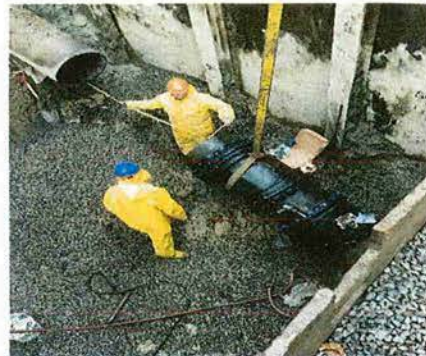
Tie in at Section 42
