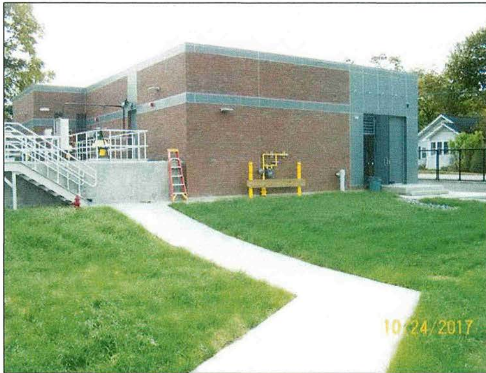
Clinton Wastewater Treatment Plant Phosphorus Reduction Facility
