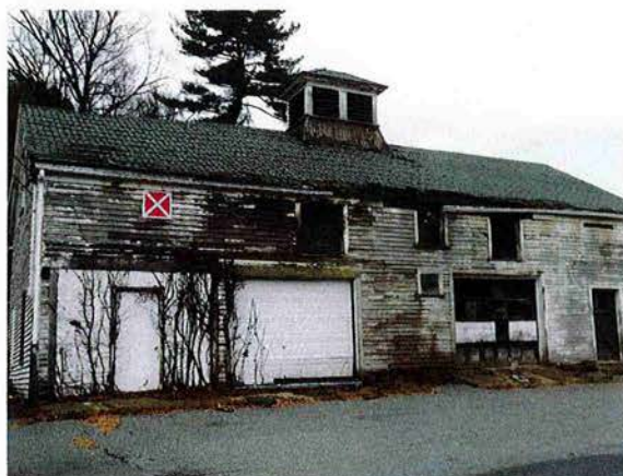
Barn behind the Oren Nichols House
