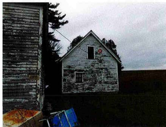
Office Storage Building
