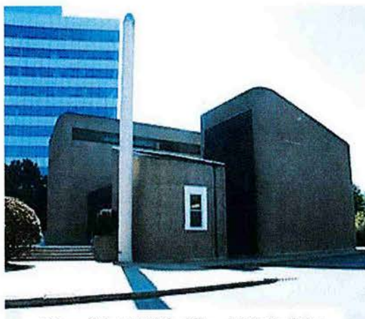
Prison Point CSO Facility – Main Building
