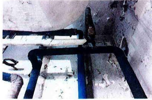
Existing piping condition concealed by insulation
