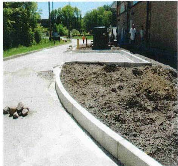
Marlborough Maintenance Facility Concrete Curb Installation
