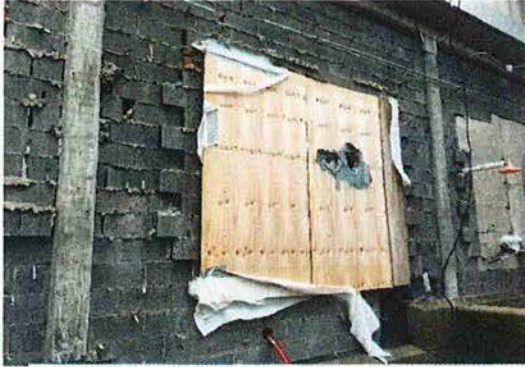
CMU of Varying Size Around Openings
