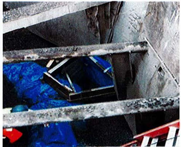
Thrust Block Formed for New MWRA 36-Inch
