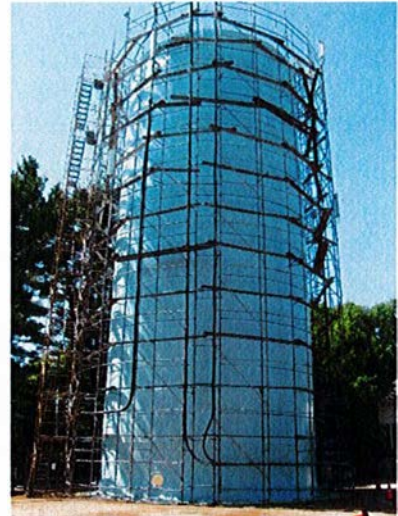
Rehabilitated Water Storage Tank
