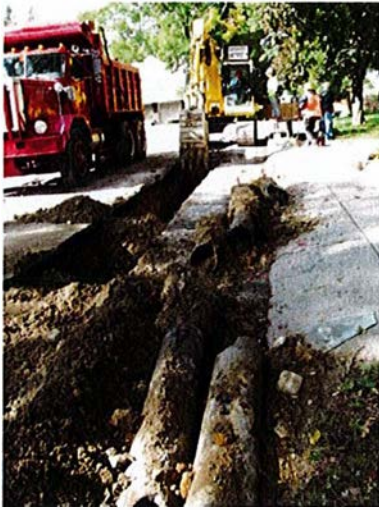
Water Main Replacement Construction
