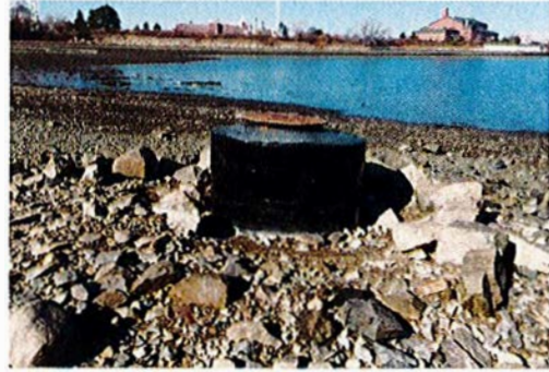
Sewer Manhole at Beach - Raised and Sealed
