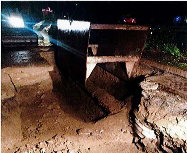
Excavation of DWWD 12-Inch Water
