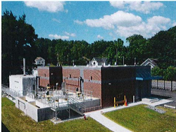
Phosphorus Reduction Facility
