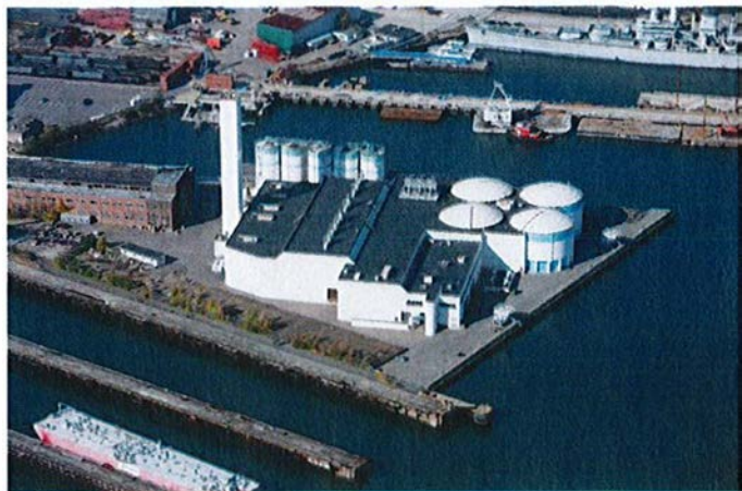
Figure 1: MWRA's Pelletizing Plant
