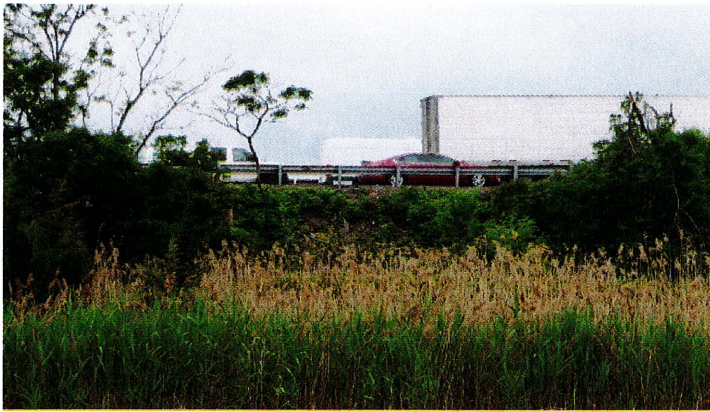
Figure 2 - Route 93 crossing near Granite Avenue, Milton
