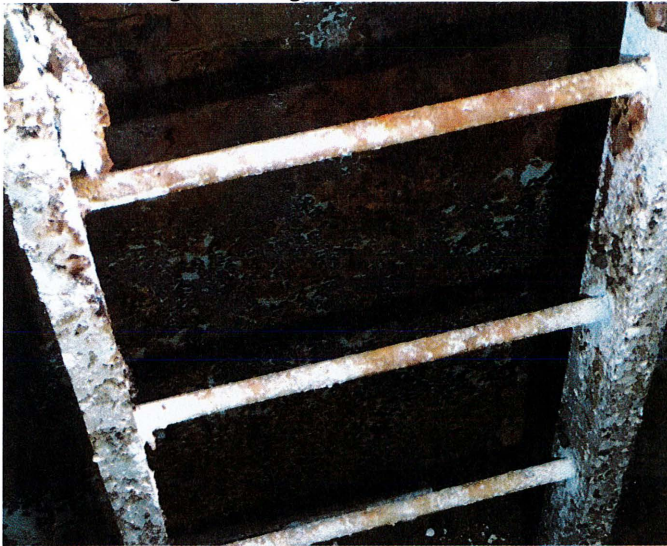
Figure 4 – Digester Overflow Box
