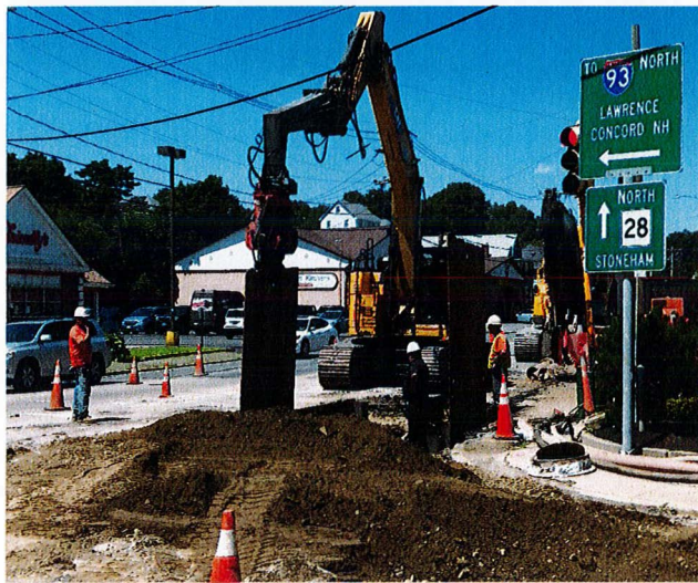
Installation of 18-inch Drain Line on Main Street
