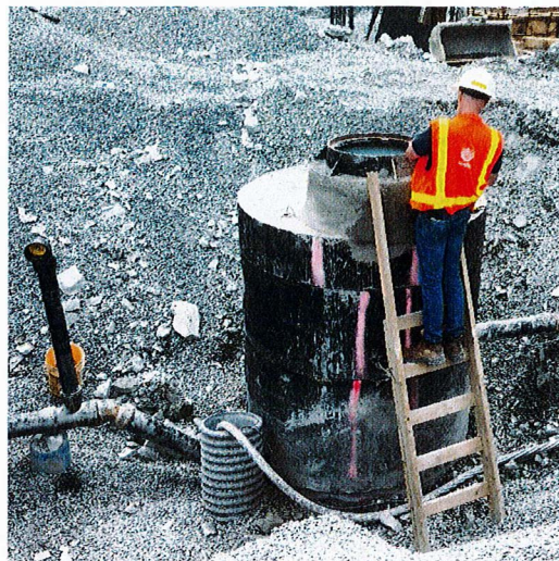
Figure 2. Inspection of a new gas/oil separator.
