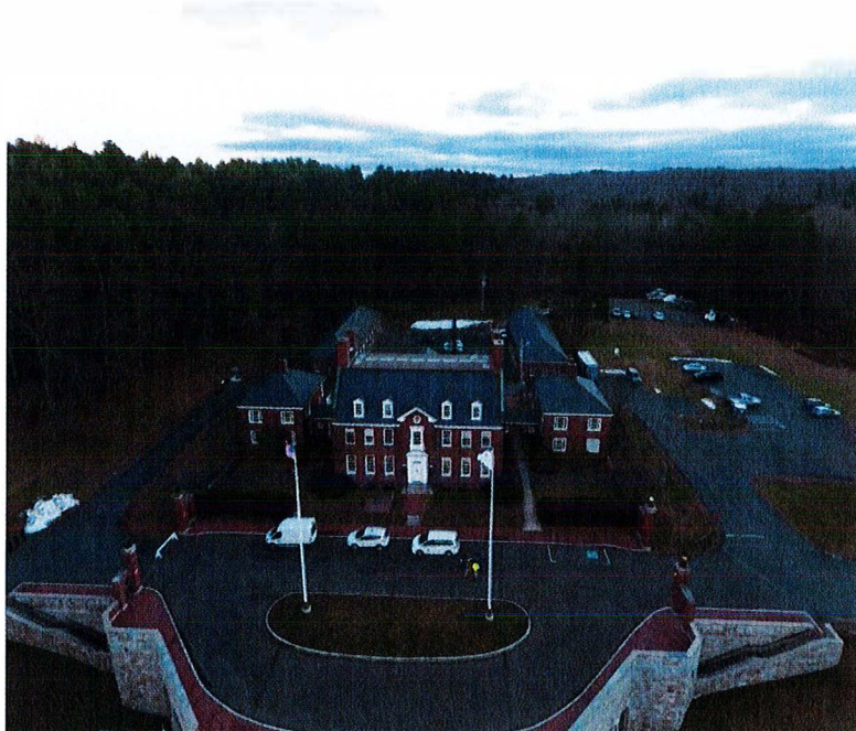
Figure 2: Quabbin Administration Building
