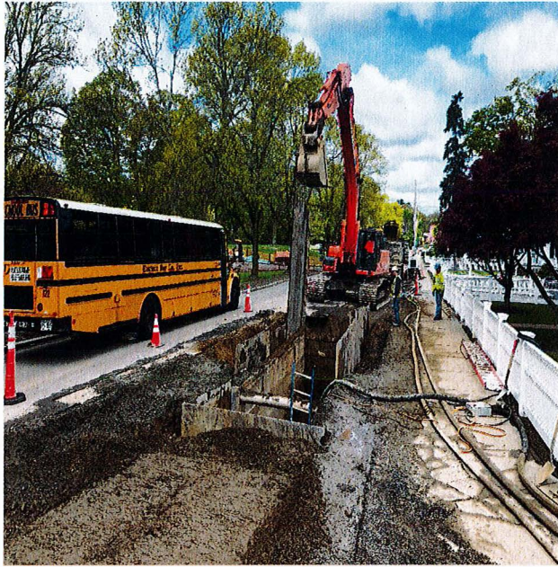
Installation of 48-inch water main on South Street
