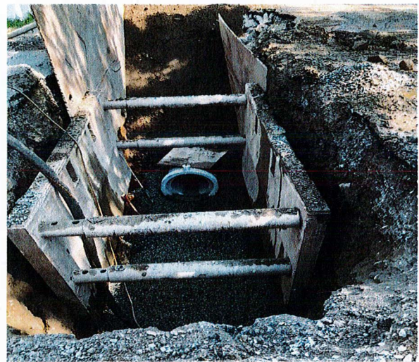
Installation of 18-inch Drain Line on Main Street
