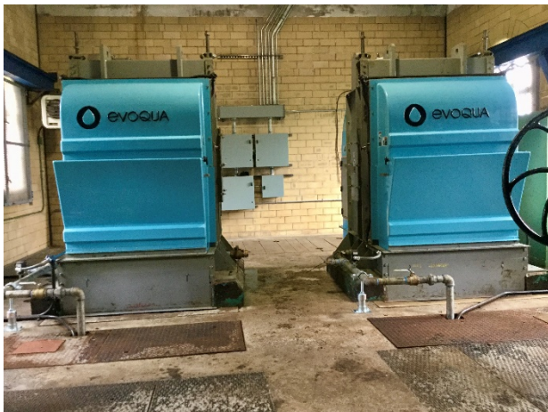
Replacement of Winsor Dam traveling screens
