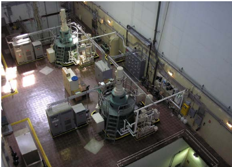
Figure 1: Cosgrove Intake Facility - Two 1.2 MW Kaplan Turbines
