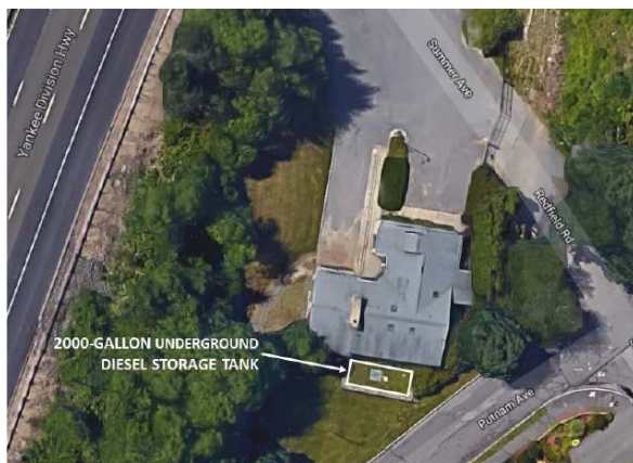
Hayes Pump Station Tank Replacement
