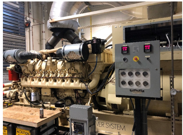
Replacement of generator alternator
