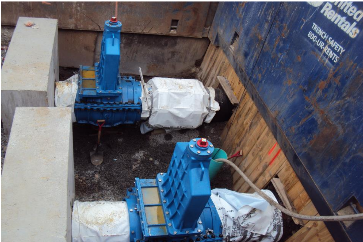
Two insertion valves installed on the existing 24-inch Shaft 6 suction mains
