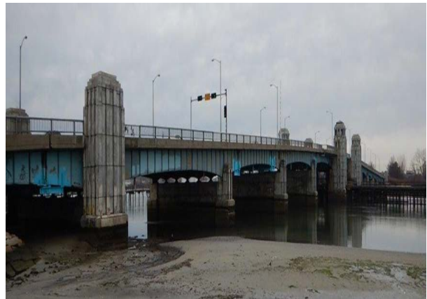
Removal of Water Main Section 56 General Edwards Bridge
