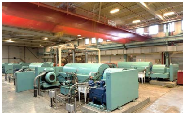
Figure 2: Dewatering Centrifuges
