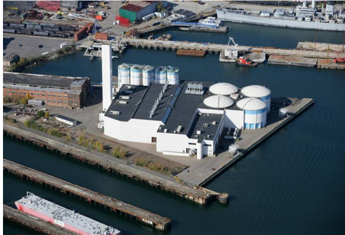
Figure 1: MWRA's Pelletizing Plant
