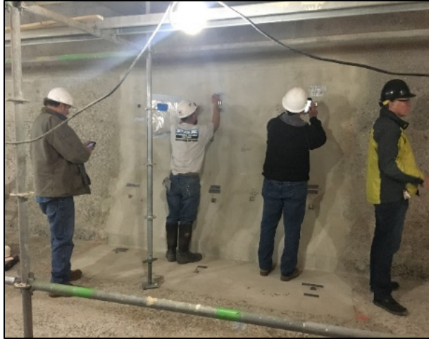
Mock-up to evaluate resurfacing products
