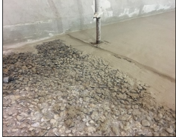
Resurfacing material applied to the channel floor
