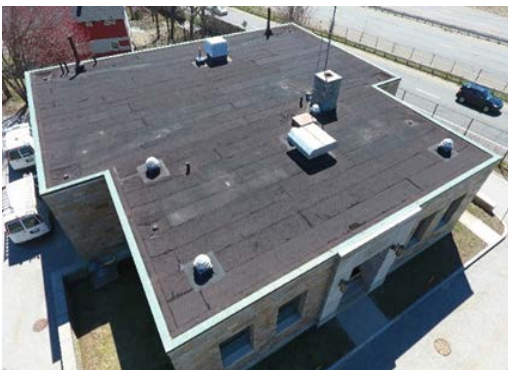
Figure 2- Spring St. Pump Station Roof
