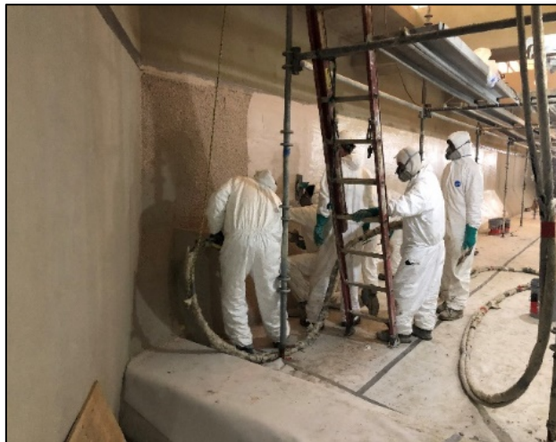
Applying resurfacing material to channel walls
