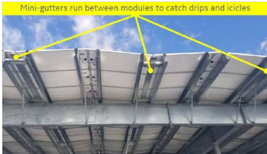
Figure 4: DSP “Mini-Gutter” System
