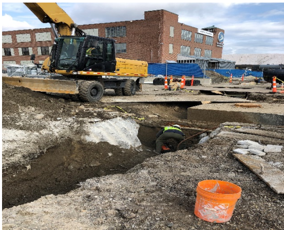
Figure 1 Crane Slab Demolition
