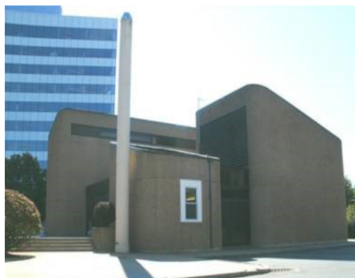
Prison Point CSO Facility—Main Building
