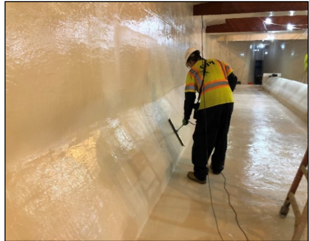
Spark testing final epoxy lining system
