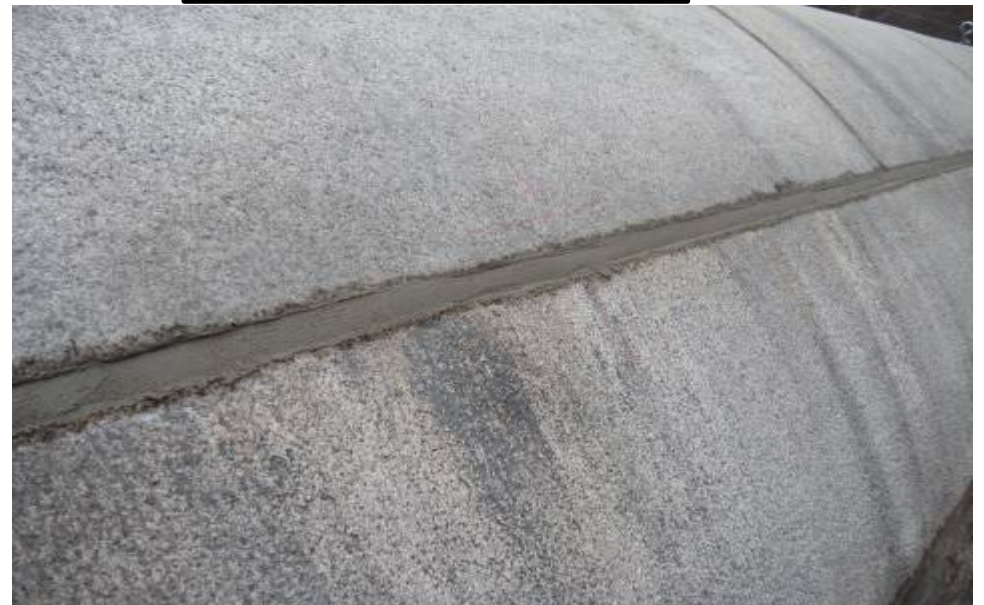
Downstream crest after
