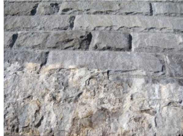
Uncleaned efflorescence
