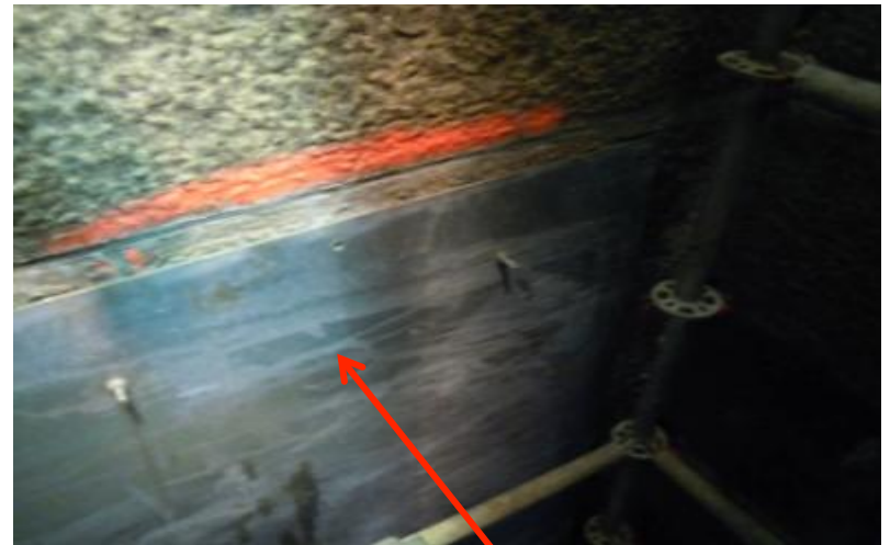
Steel plate for protection against erosion of mortar
