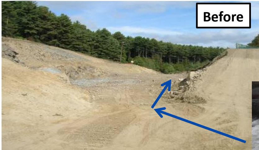
Spillway Constriction
