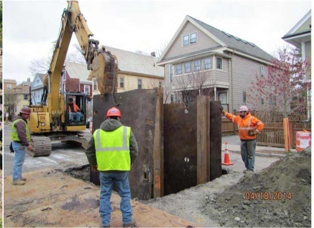
FY16 Marks the Completion of CSO Program Construction June 3, 2015
