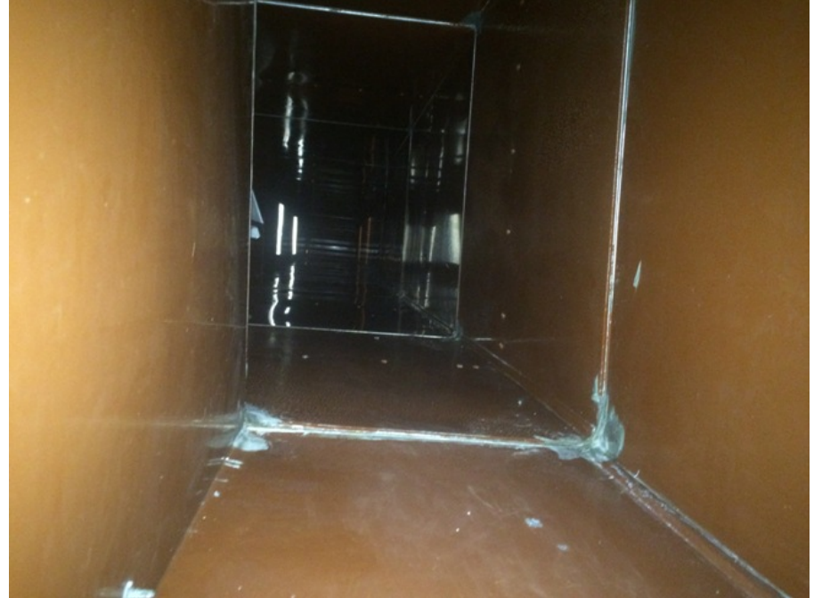
Cleaned Ductwork
