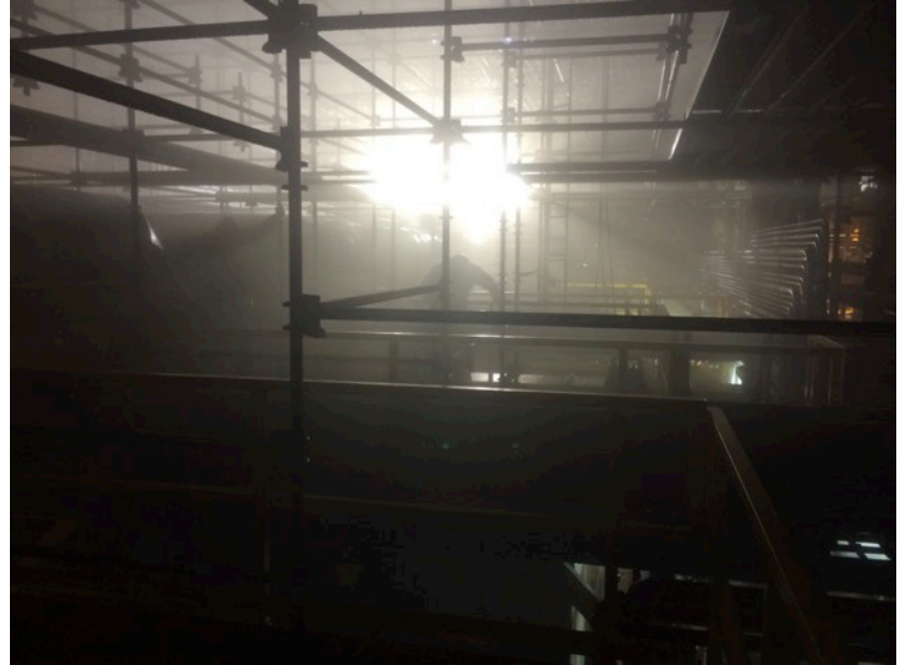
Significant Staging Effort
