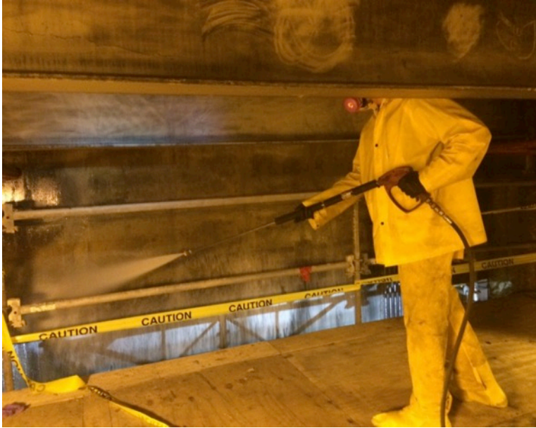
Power Washing Upper Beams
