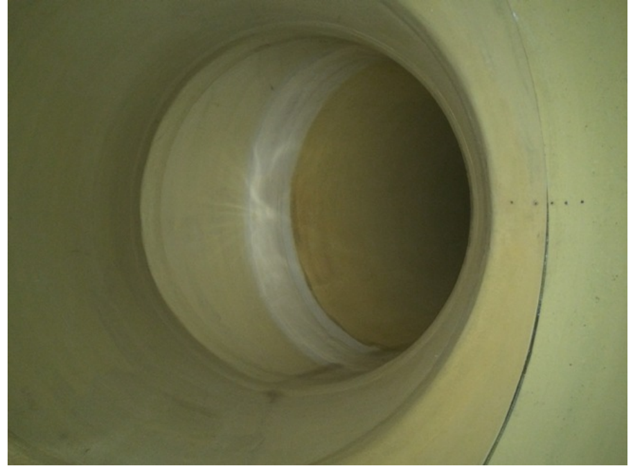
Cleaned Ductwork
