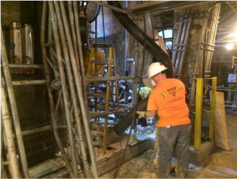
Vactoring Media Balls from Scrubbers
