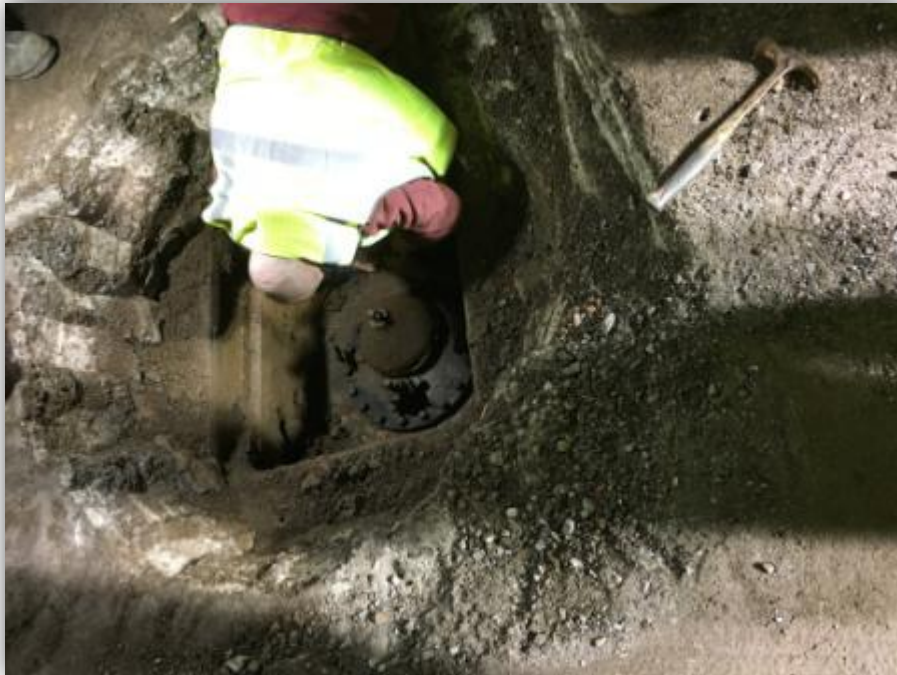
Air Release Valve assembly installed on existing pipe 4/2, 11:55 P.M.
