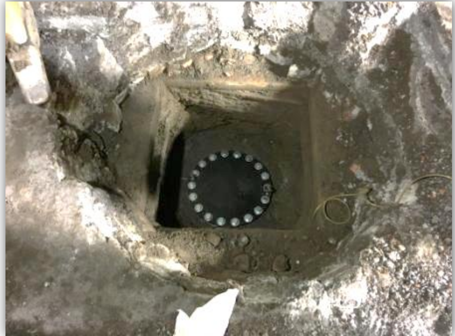
New Flange Plate installed 4/3, 12:40 A.M.
