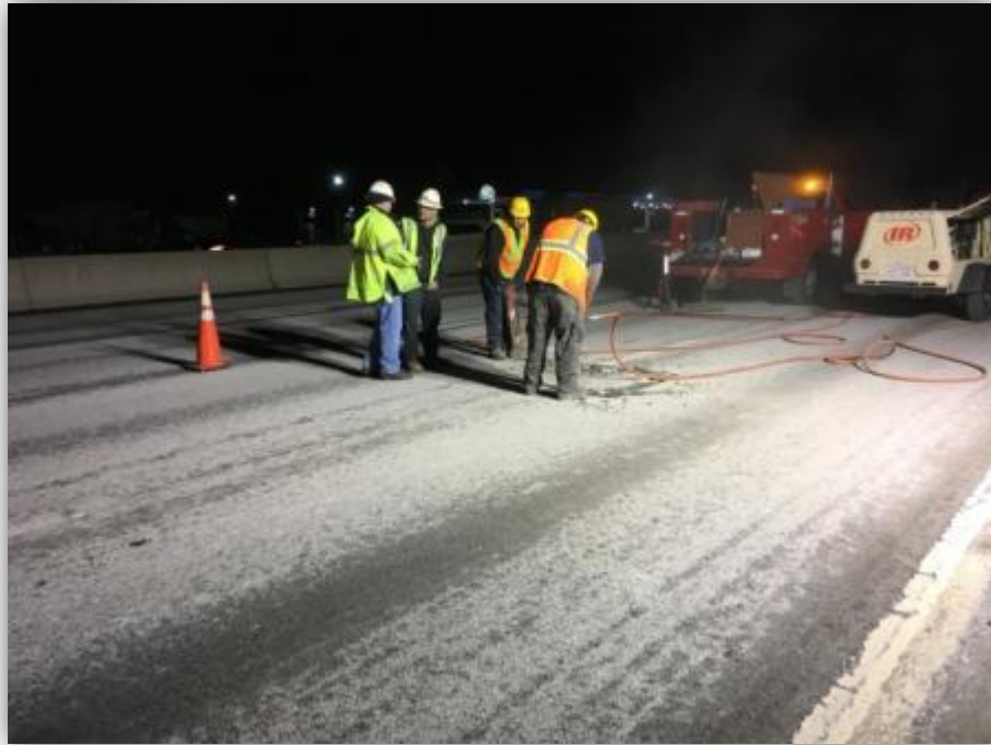
Cutting pavement in lane 4/2, 10:15 P.M.
