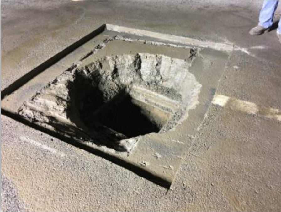
Prepared Trench 4/3, 1:20 A.M.
