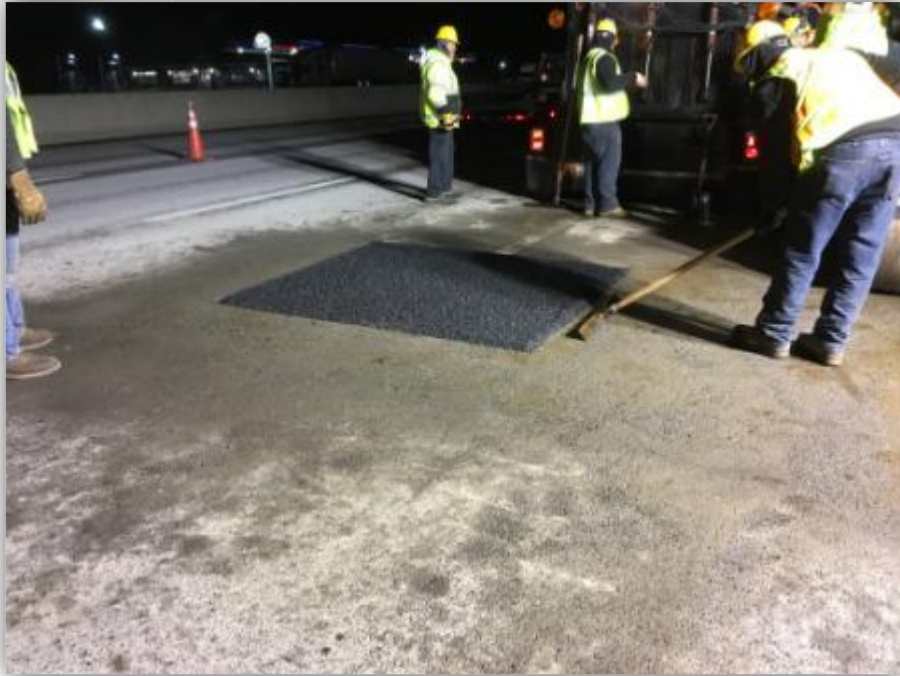
Temporary Trench paving 4/3, 2:40 A.M.
