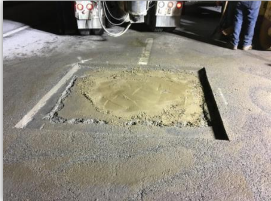
Backfilled with CDF 4/3, 1:30 A.M.
