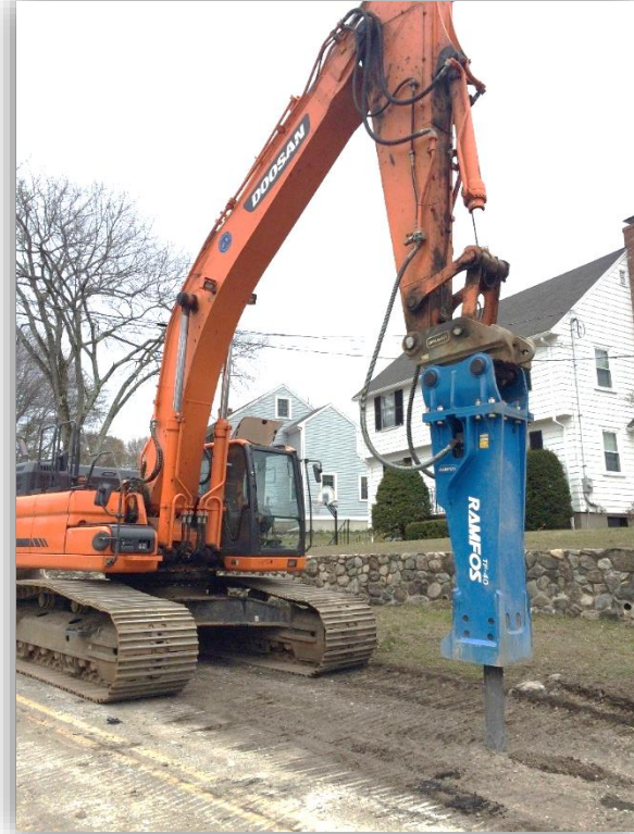
Hydraulic ramming of ledge
