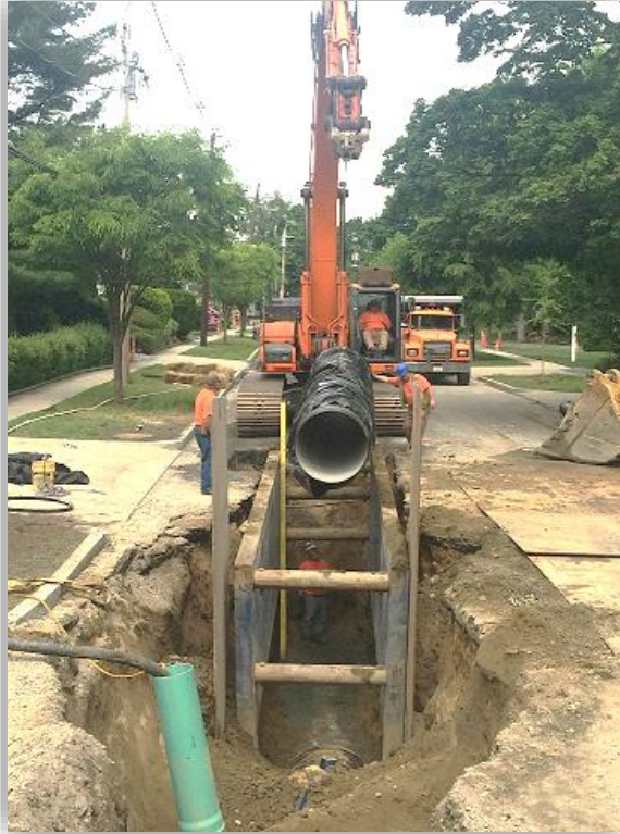
Installation of 36-inch DI pipe on Summer Ave
