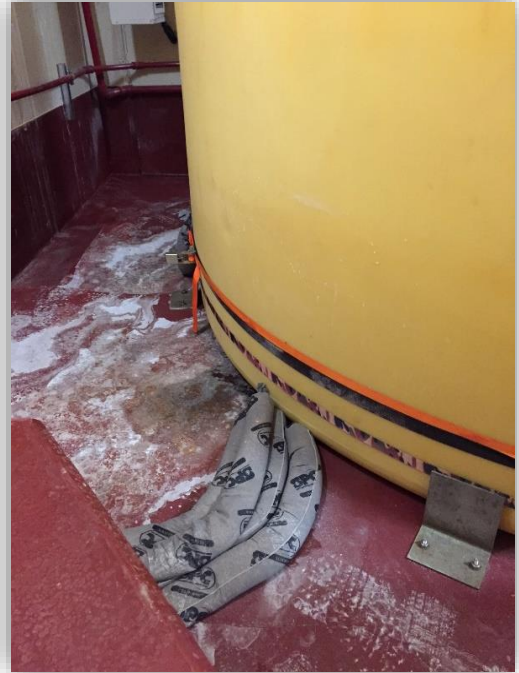
Replacement of Leaking Chemical Tanks
