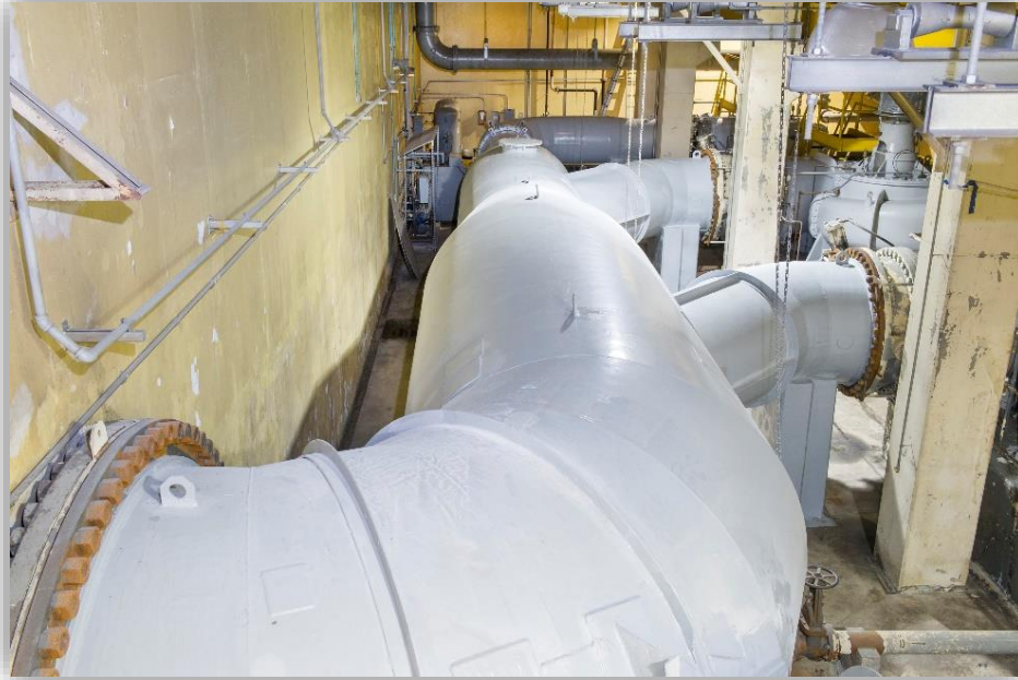
Interior Lining of Wet Weather Discharge Piping
