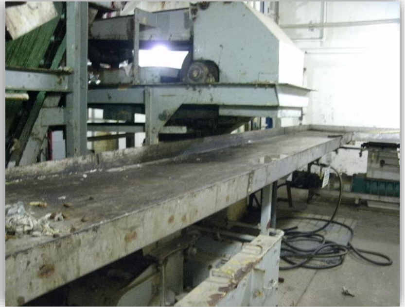
Replacement of Conveyor System
