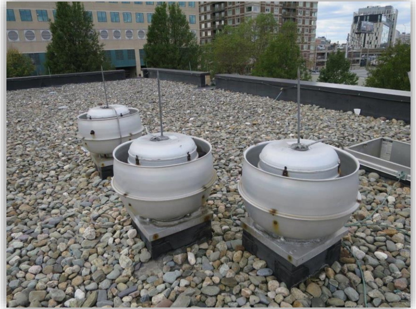
Replacement of Lightning Protection on Chemical Building
