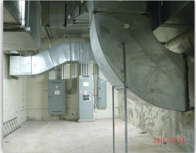
Relocation of Electrical Room
