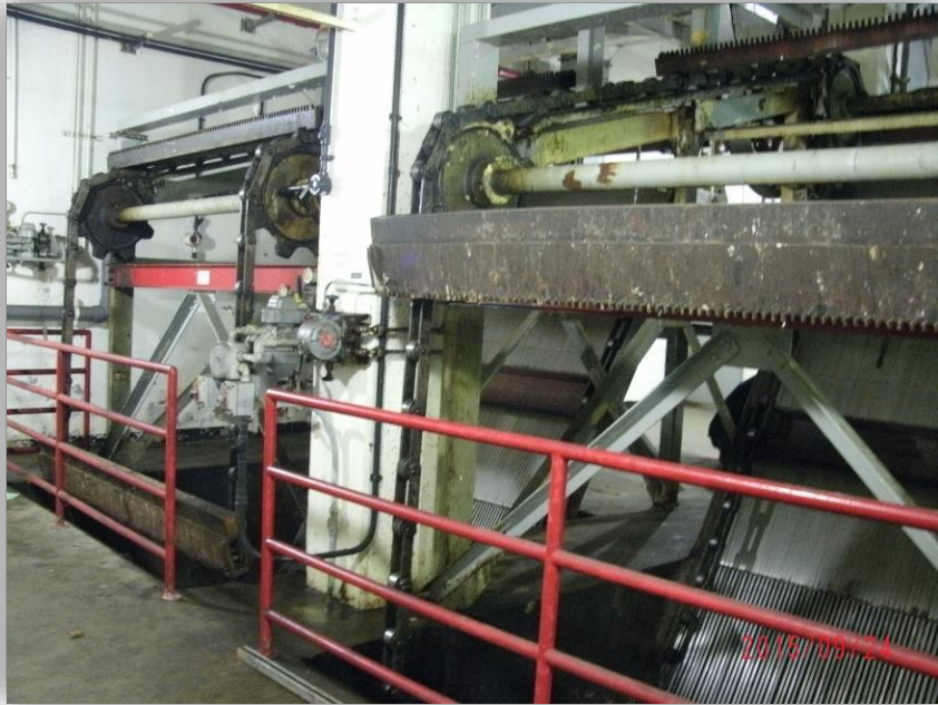
Mechanical Bar Screens to be Replaced
