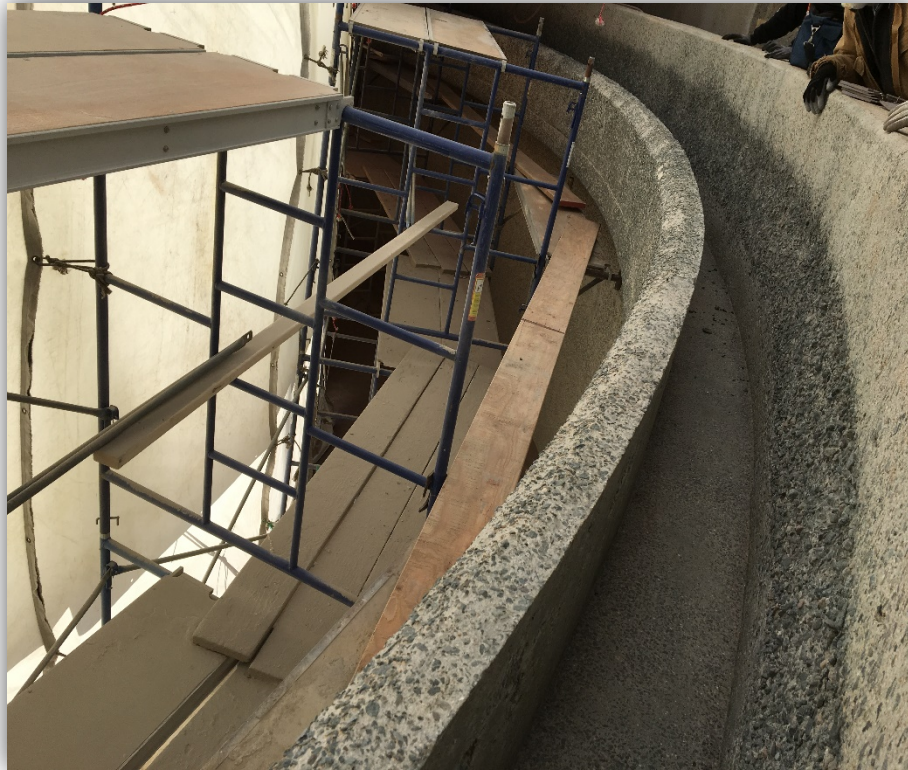
Existing Interior GT Walls
