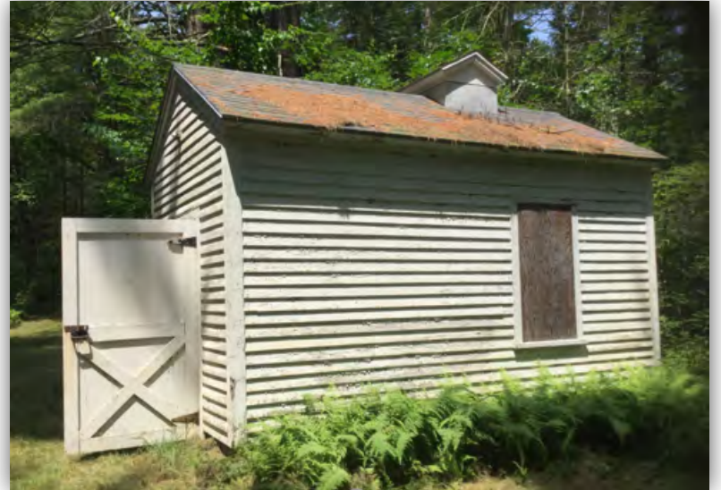
Well Pump House
