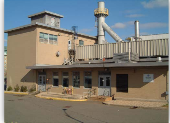
Ward Street Headworks
