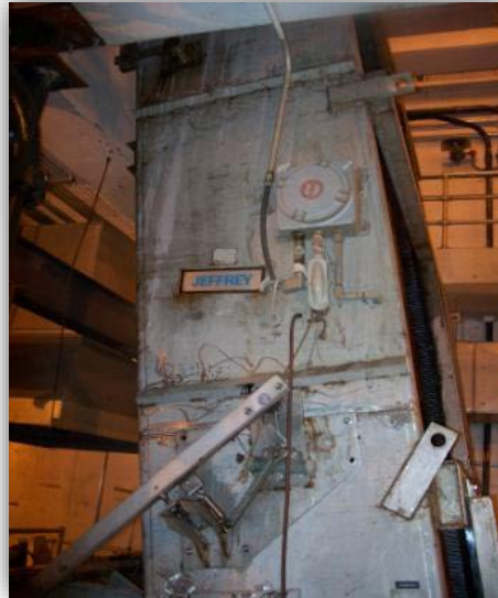
Climber screen replacements
