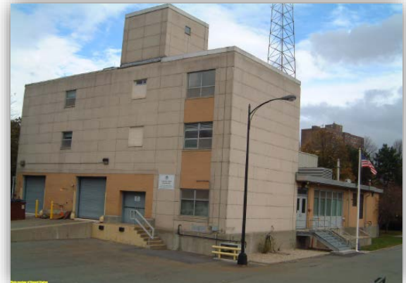
Columbus Park Headworks
