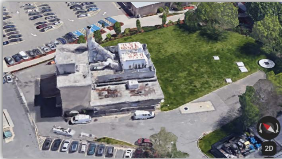
Existing Ward Street Headworks Facility
