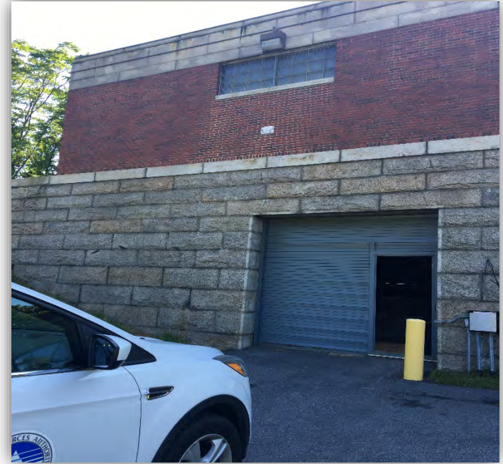
Shaft 5 - Front View
