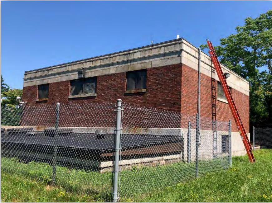
Shaft 5- West/ Rear View
