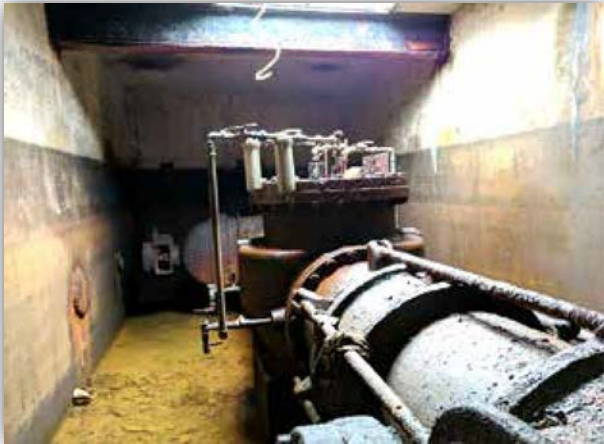
W16 Nonantum Road Vault and PRV (existing)
