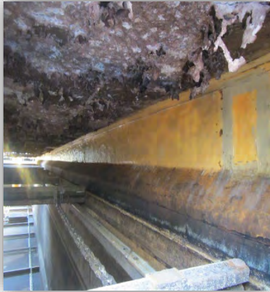
Coating Failures
