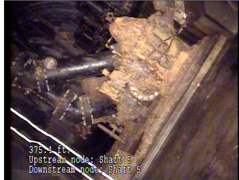
Underground pump room (abandoned with fill)
