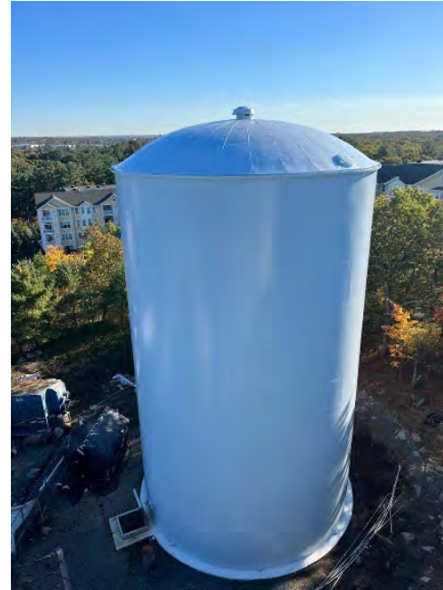
Water Storage Tank Rehabilitation
