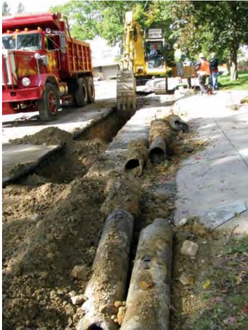
Water Main Replacement Construction
