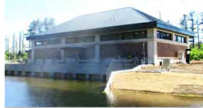
Wachusett Aqueduct PS – Geothermal Heat Pump
