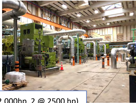
4 Large Air Compressors (2 @ 2,000hp, 2 @ 2500 hp)
