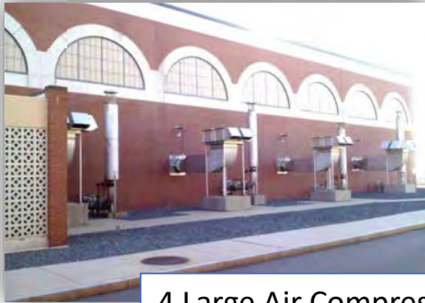
4 Large Air Compressors (2 @ 2,000hp, 2 @ 2500 hp)
