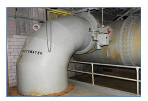
Thirty feet below this is valve #2. Both get replaced. We will cut the pipe at the elbow and remove the valve in the first outage at each valve. This is the most critical shut-down and replacement. The replacement will include a flange (the original is not), so that next time we have to replace the valves the pipe is bolted, not soldiered.
